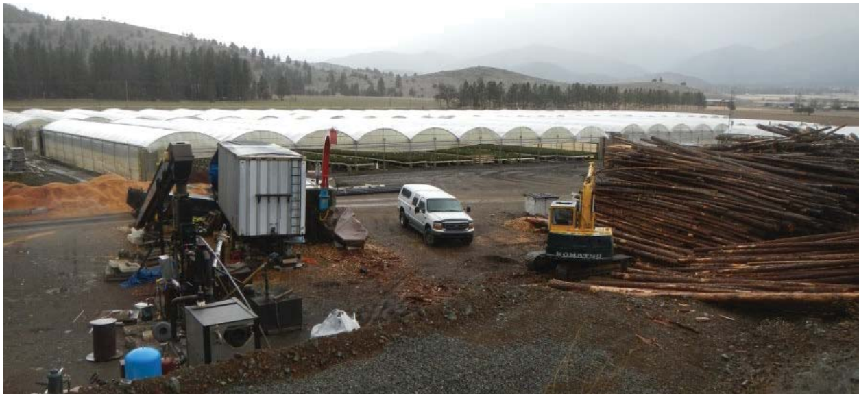
Wood gasification system heats greenhouses at CalForest Nurseries utilizing wood fuel chips produced as a by-product of thinning operations to improve forest health.
