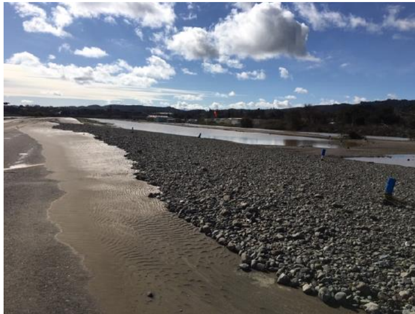
FIGURE 10-19: CLOVERDALE AIRPORT RUNWAY FLOODING, FEBRUARY 2019
