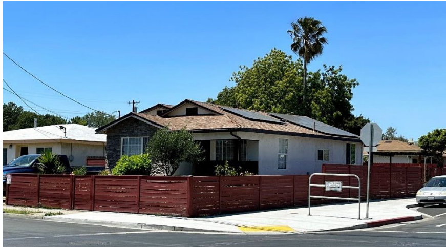
Solar panels help reduce reliance on natural gas and electricity providers and increase resilience for homeowners.
