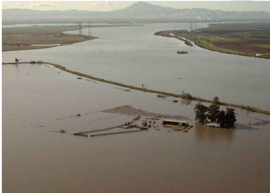
Delta flooding, as occurred on Bradford Island in 1983, is a significant hazard in Contra Costa County. (Credit: California Department of Water Resources)
