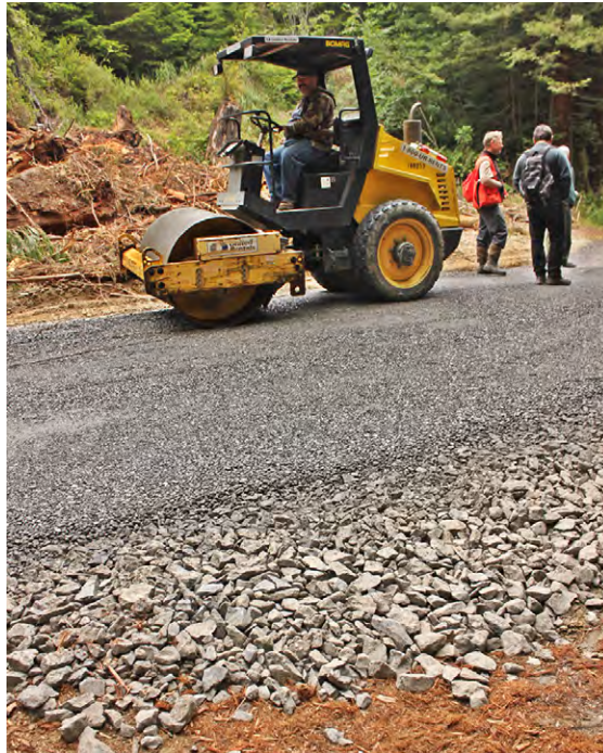
FIGURE 170. Road structural cross section showing a gravel surface course bound by finer material, overlying an angular base course spread and compacted on a stable, natural subgrade.
