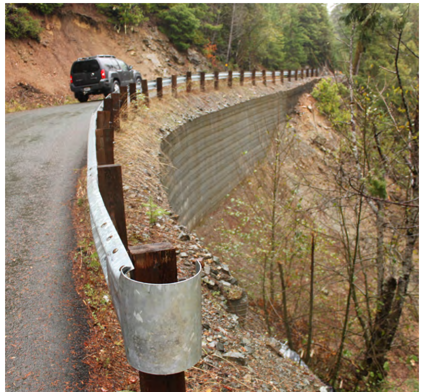
FIGURE 212. Engineered fill constructed where a fill slope failure had removed the entire roadbed.
