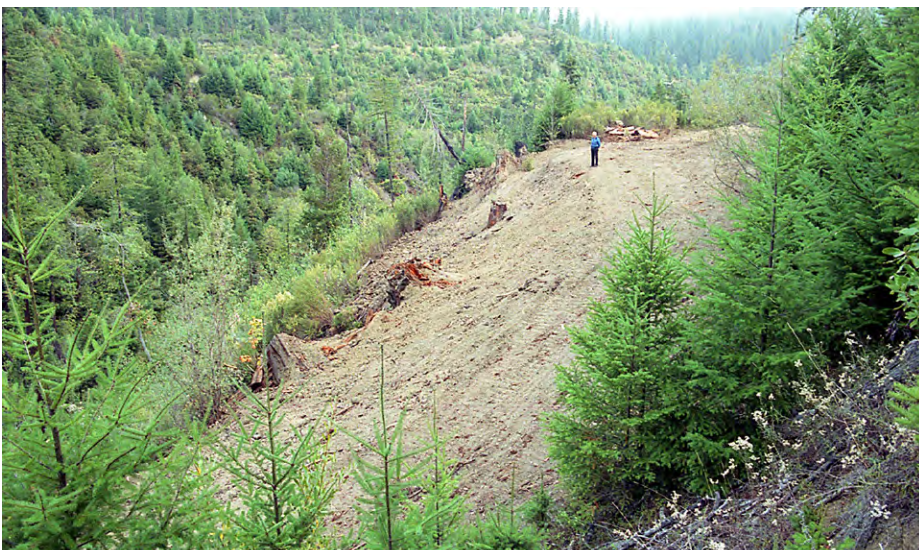
FIGURE 273B. The excavation required a temporary road be built across the middle of the long fill slope to reach all the unstable material. The concave excavation surface mimics the shape of a potential slide plane and thereby assures that most of the unstable fill material has been removed. Spoil materials were pushed up against the inside of the large landing, entirely on a stable, excavated bench as in Figure 272B. This type of outsloping is called an “Inplace Outslope” (IPOS), where all the excavated materials were stored locally (note person for scale).
