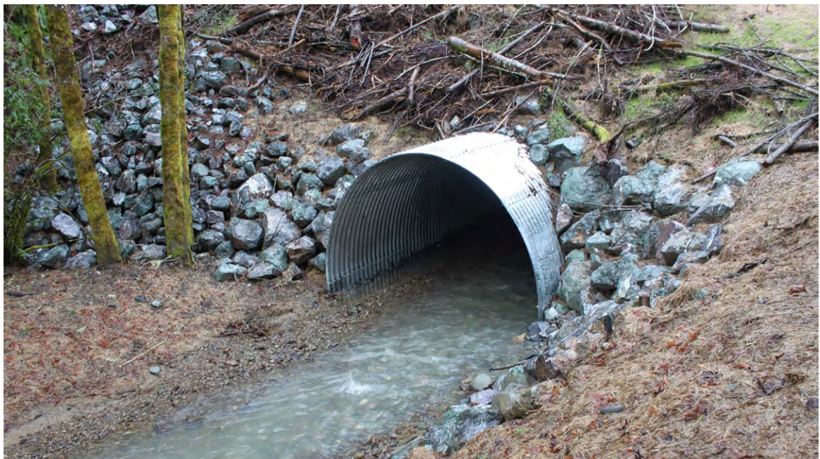
FIGURE 73. Embedded culverts are another type of stream crossing structure that allows continuous fish passage. This 10-foot diameter embedded culvert has a natural gravel and cobble streambed. It was installed to replace a small diameter culvert that was a barrier to fish migration.
