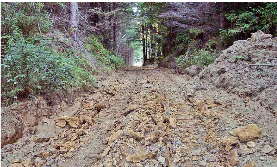
FIGURE 278B. A road after ripping and decompaction.
