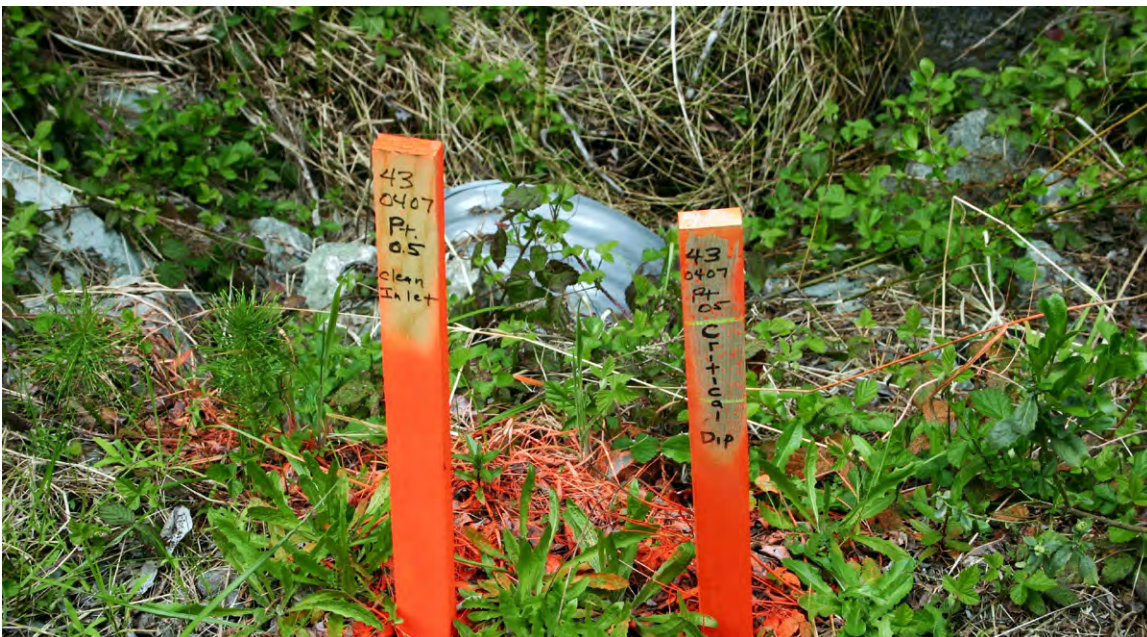
FIGURE 236. For large landowners, maintenance tasks can be identified on a data form, and staked on the ground by inventory crews. This small stream crossing needs a critical dip to prevent future stream diversion, and the inlet needs cleaning; tasks to be completed by maintenance crews or contractors.
