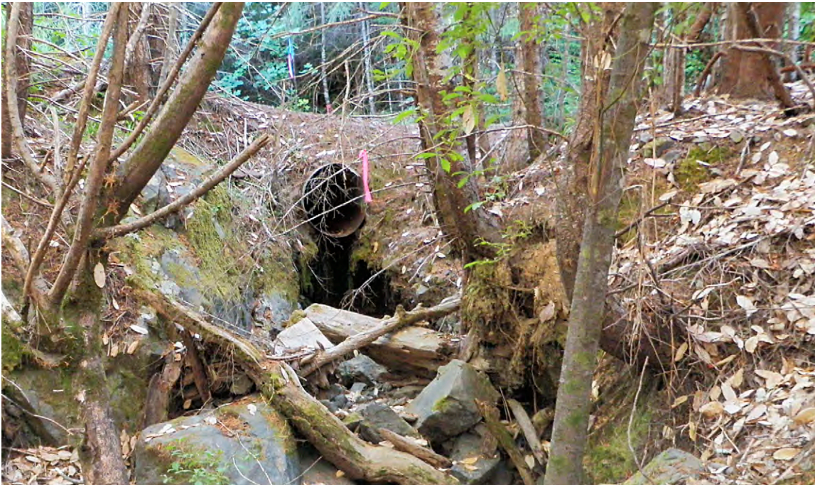
FIGURE 217A. Culverted stream crossing on a permanent forest road before upgrading to the 100-year design standard (including debris and sediment). The before and after photos of the culvert outlet are taken from the same location.
