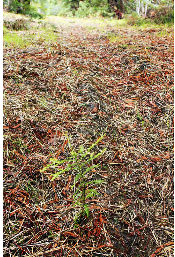
FIGURE 283. Tree planting (or planting woody species suitable for the specific environment of the road) is the final long term treatment for the decommissioned roadbed and for the riparian sideslopes where stream crossings have been excavated and restored for the long term. This planted redwood tree, and those conifers and hardwoods that naturally seed themselves onto the former roadbed, will eventually cover the alignment and provide for long term site stability.
