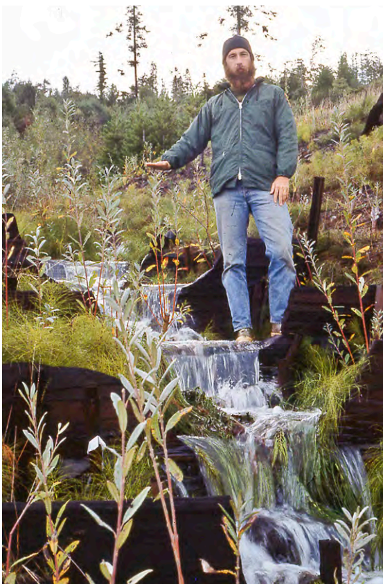
FIGURE 180. Board check dams constructed in a gully to prevent downcutting and stabilize the bed and banks. Willow cuttings planted and growing in the bed and banks will eventually stabilize the gully once their roots are well developed.
