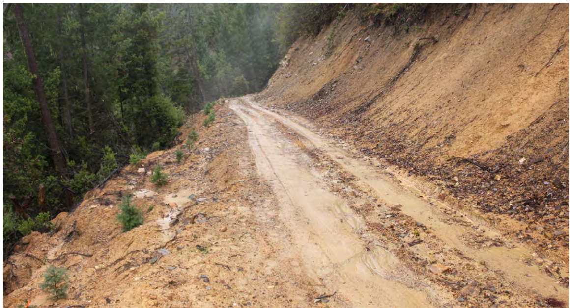
FIGURE 143. Sidecast road construction on steep inner gorge slopes above a fish-bearing stream. Fine grained sidecast materials are perched on 70% slopes and show signs of instability and pending failure. The remaining, stable part of the roadbed is on the road cut.
