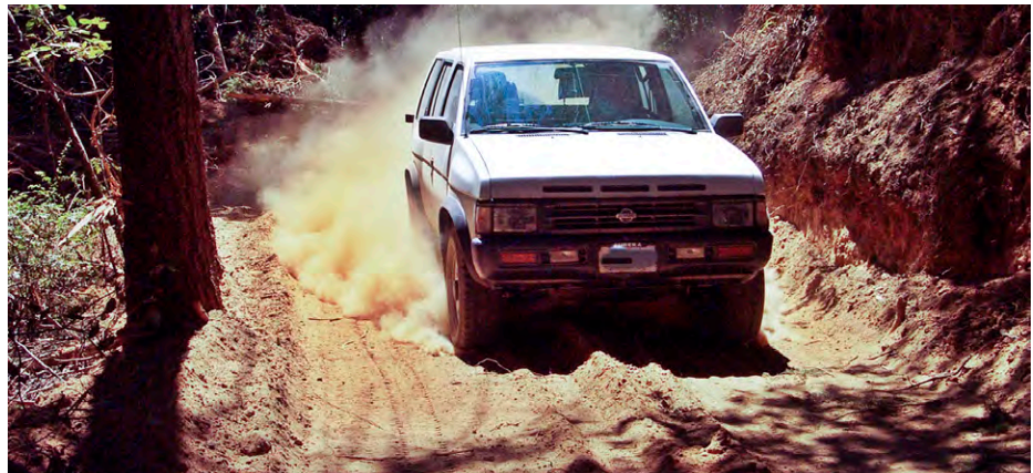
FIGURE 248 A & B. Excessive road dust during the summer (248a) and excessive mud during the winter (248b) are conditions which directly threaten water quality and result in high road maintenance costs. Both conditions produce and deliver large quantities of fine sediment to nearby streams during periods of surface runoff. This fine material can be especially damaging to fish and fish habitat.
