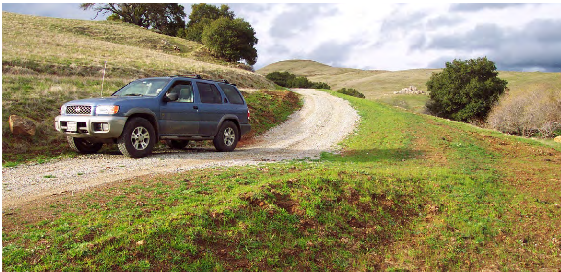
FIGURE 224B. The same road after being converted to an outsloped road with rolling dips to improve road drainage and decrease maintenance requirements and costs. The road was also gravel surfaced so it could be used during wet weather periods.
