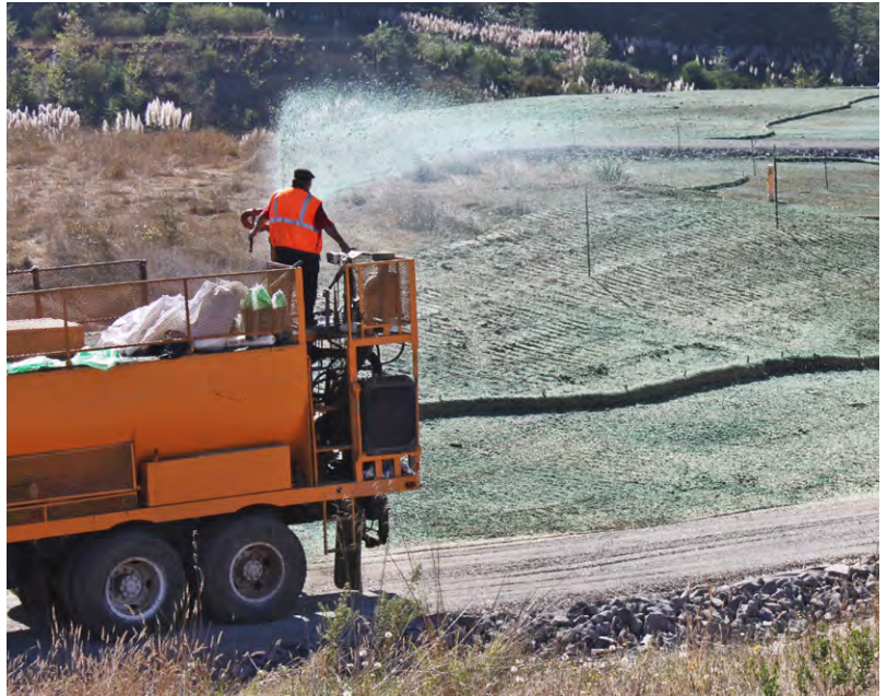
FIGURE 282. Hydroseeding (spraying a slurry of water, mulch, seed and fertilizer) on bare soil areas can be an effective erosion control and revegetation treatment for large disturbed areas, or for bare soil areas along open roads. It is most useful for treating spoil disposal sites, after they have been graded and smoothed, and for treatments along newly upgraded roads where the truck or trailer can have easy access. Hydroseeding decommissioned roads is more difficult because access is cut off as the treatments progress. Rather, hand seeding and mulching is usually the preferred treatment.
