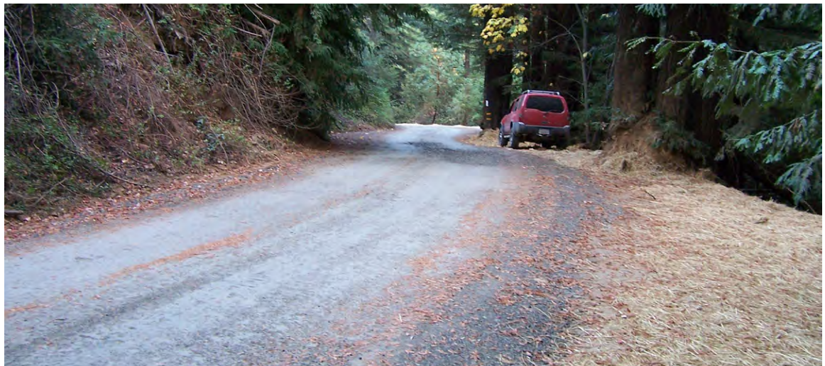
FIGURE 225B. The same road was converted to a gravel surfaced outsloped road with no inside ditch or outside berm (b). The shoulder has a steeper outslope to provide for free, continuous drainage of road surface runoff.
