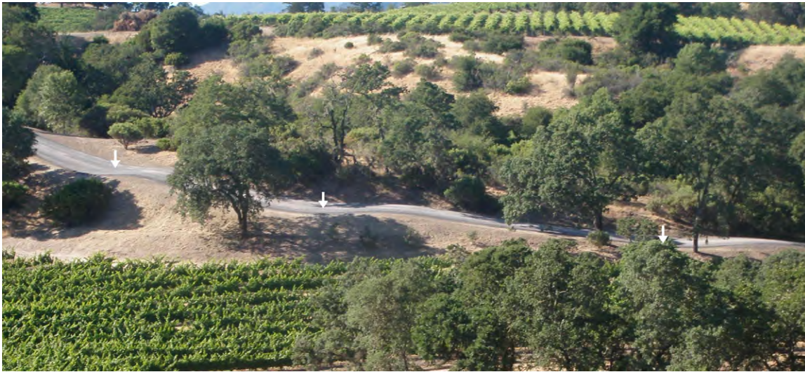
FIGURE 38. Rolling dips should be spaced on outsloped roads so that the road surface is well drained and free from erosion, and the slopes below each dip show minimal erosion. Three broad rolling dips (see arrows) are visible in this upgraded road reach used by both commercial and residential traffic.
