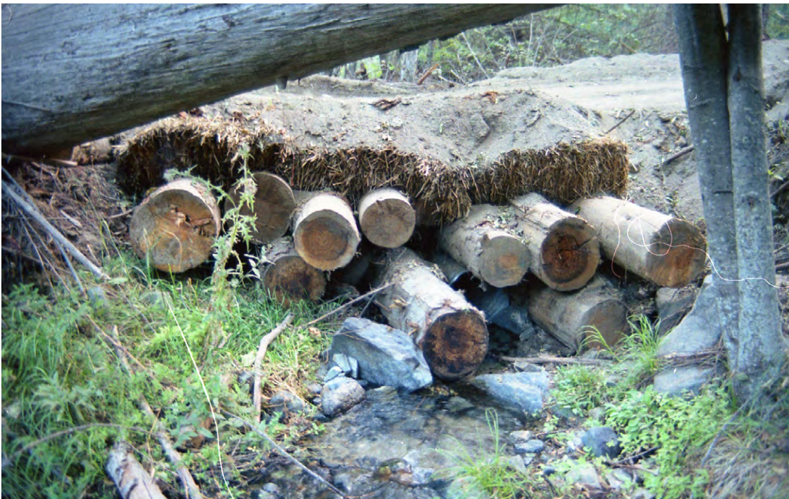
FIGURE 126. This small, temporary log crossing is constructed with a culvert at its base, with logs, straw bales and finally road surfacing material on top. A geotextile fabric can be used instead of straw to provide separation between the stream and the overlying road materials. Ideally, the road surfacing materials should be clean road rock or gravel (not dirt) that will not adversely affect water quality if some makes its way into the stream. Temporary crossings should be removed before each wet weather season.
