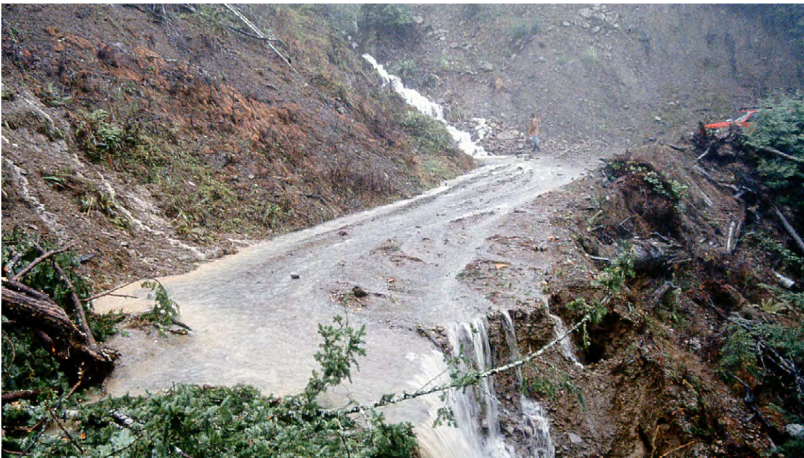
FIGURE 2. This stream crossing “washed out” (eroded) when the culvert plugged and streamflow overtopped and scoured through the road fill. Sediment was delivered directly to the stream system as the fill eroded. Stream crossings and culverts need to be properly designed, constructed and maintained to minimize the potential for such failures.
