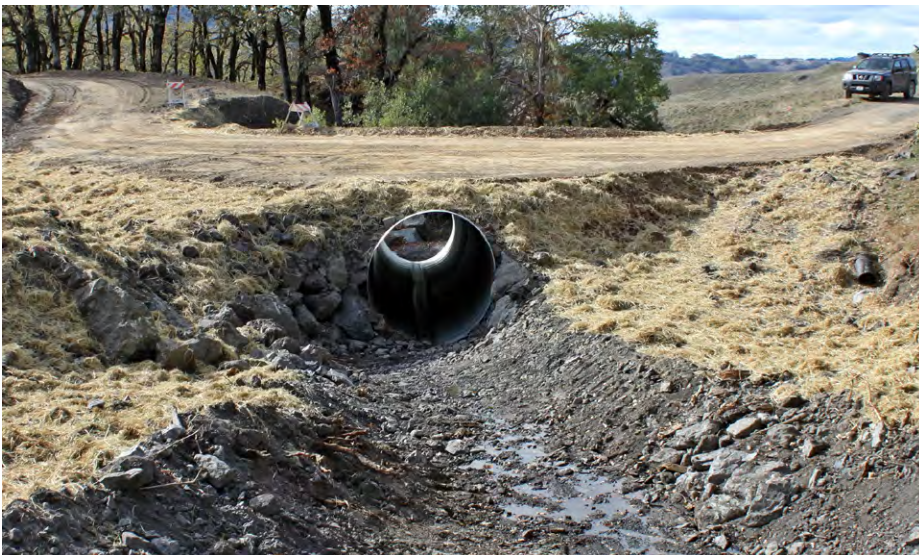
FIGURE 157A. Culvert installation in a shallow fill on a steep, boulder bedded Class II (non-fish bearing) stream replaced a severely undersized pipe (Figure 157a). The new six foot diameter culvert is set slightly into the original streambed and the inlet is armored to prevent erosion. The aggraded channel above the inlet (foreground) has been excavated and disturbed bare soil areas have been mulched and seeded. The roadbed dips into and out of the stream crossing with a critical dip placed just down-road of the left hinge line.
