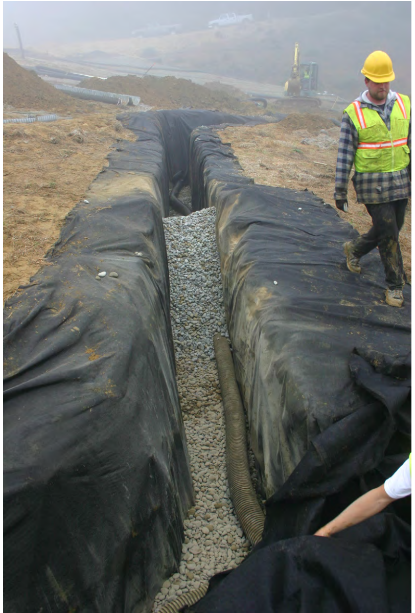
FIGURE 142. Pipe underdrain used to capture subsurface groundwater before it can saturate an adjacent fill slope. This trench was 10 feet deep and 2 feet wide, lined with non-woven geotextile and filled with gravel. A perforated flex pipe was placed on a thin layer of gravel at the bottom of the trench and the drain sloped gradually downhill and discharged captured subsurface flow onto a nearby stable slope.
