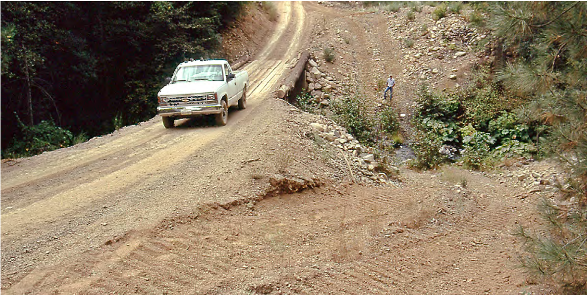
FIGURE 148. Many bridges built on small forest and ranch roads cannot support or would be damaged by heavy tracked equipment passing over them. For this reason, an adjacent equipment ford is sometimes constructed. These steep fords can erode and deliver sediment to the stream channel if they are not rock surfaced, or waterbarred, mulched, and seeded between uses and prior to the rainy season.
