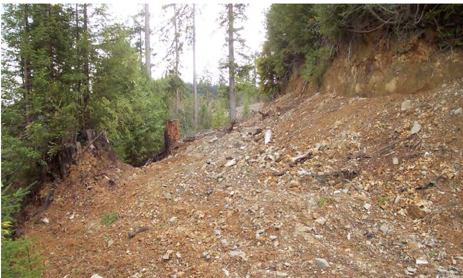
FIGURE 270B. Spoil excavated from the nearby unstable fill slope was hauled to this section of road and placed (and compacted) against the cutbank. This type of treatment is called an “Import Outslope” (IOS), where most of the fill used to outslope the former roadbed was imported from another, nearby excavation site. Using local spoil disposal sites, provided they are suitable, can save significantly on endhauling costs.
