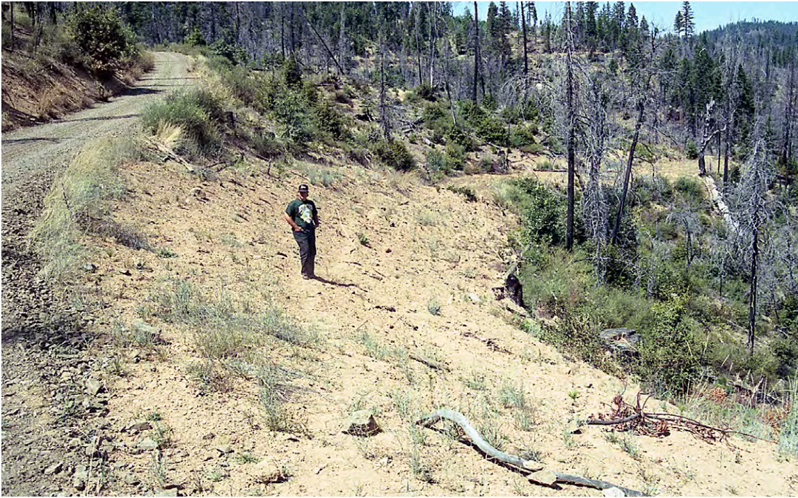
FIGURE 286. Severe outslipping, which prevents vehicle access, should only be used on temporary roads and decommissioned roads where all stream crossings have first been removed, unstable fill slopes have been excavated or stabilized, and road surface drainage is permanently dispersed. To help ensure vehicles do not use the closed road, logs, boulders and brush can be spread over the surface, especially near the beginning of the road, to discourage unwanted traffic. These roads should need no future maintenance, so vehicle access is no longer needed.
