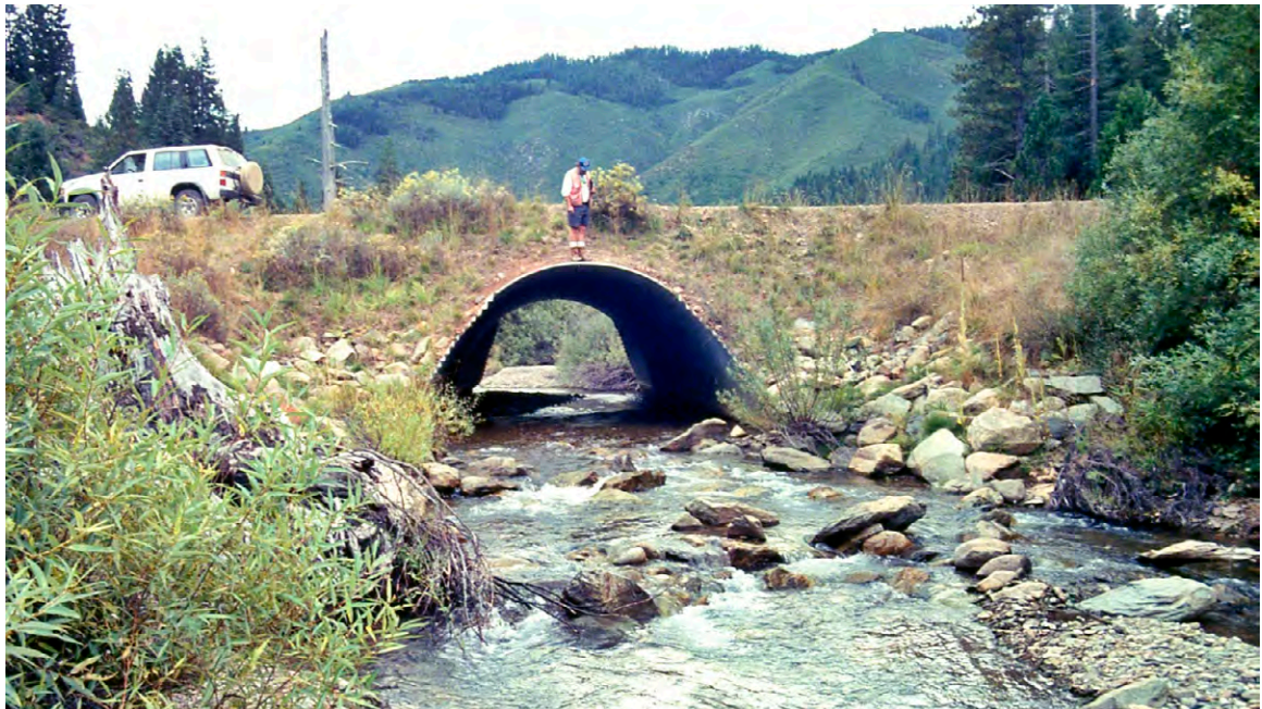
FIGURE 72. This bottomless plate arch was installed to provide fish access through the stream crossing. Each abutment is comprised of a concrete foundation and the stable stream-bed ensures continuous aquatic passage.
