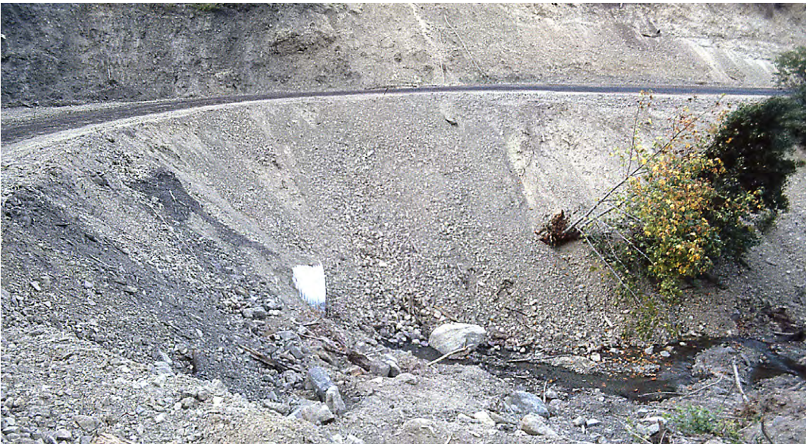
FIGURE 147. Uncontrolled sidecasting on the approach to this poorly constructed stream crossing delivers sediment directly to the stream channel. Roads built next to streams should be full bench endhailed, fill slopes should be at a stable angle (about 2:1), armor should be placed around the culvert, culverts should be extended approximately 6 feet beyond the base of the fill, and the slopes should be mulched and vegetated.
