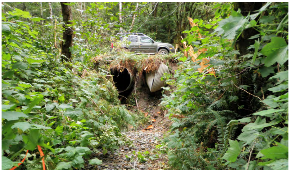
FIGURE 267A. Dual, undersized, elevated culverts at this small stream crossing have been a barrier to fish passage since the road was built decades ago. The outlet of the culvert on the right has been crushed closed, probably by heavy equipment performing maintenance work. Road and stream crossing decommissioning was used to permanently reopen the channel to fish passage.
