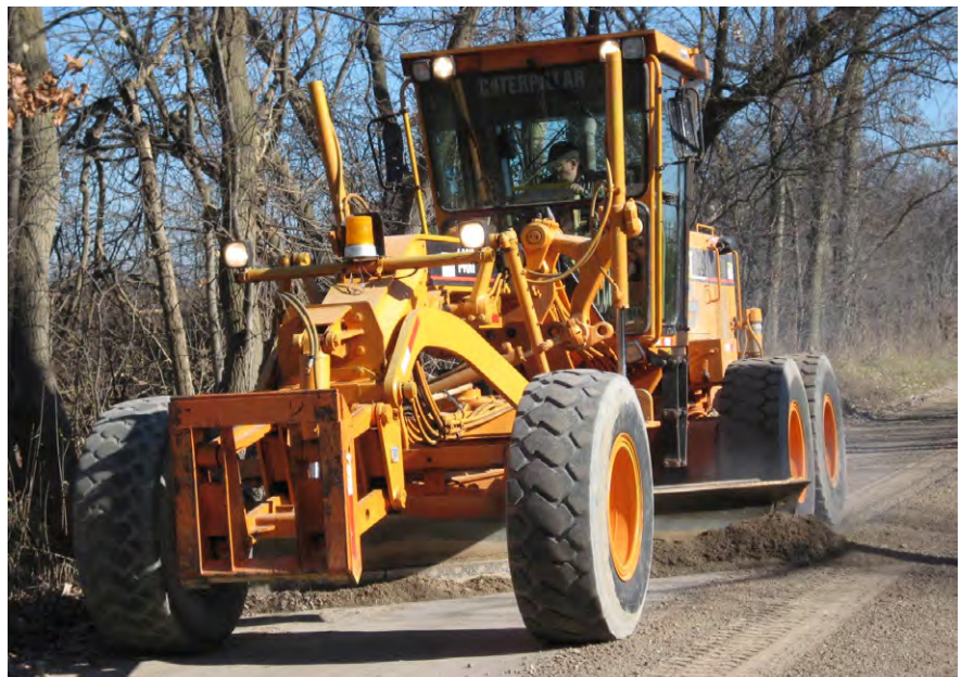
FIGURE 242. Grading a road to make a smooth running surface is beneficial for traffic, but it may also be treating the symptom of the problem rather than the cause of road roughness. Grading should have the dual purpose of 1) providing for a smooth running surface and 2) maintaining or improving road surface drainage. Grading for drainage will lower maintenance costs, as grading won't be needed as frequently. Grading only to produce a smooth road surface is a recipe for developing the exact same road problems that caused you to call for a grader.
