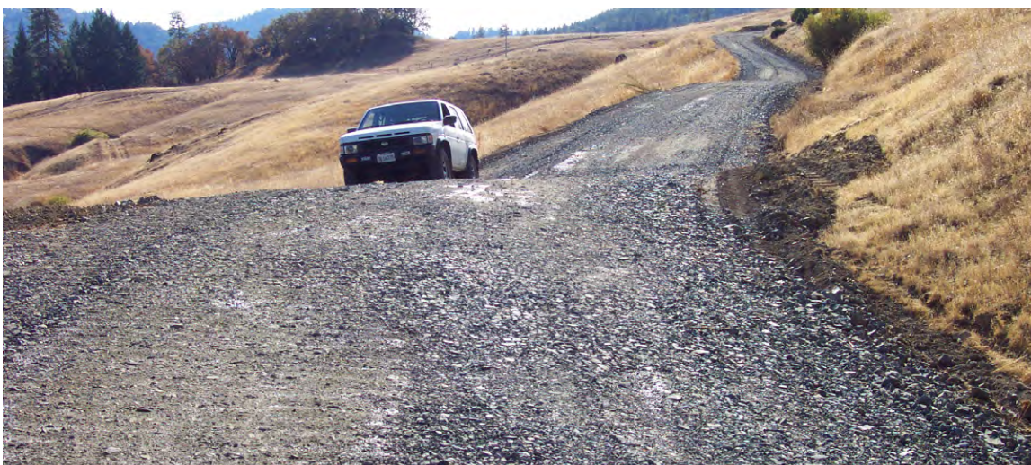
FIGURE 226B. The same road was converted to an outsloped shape, with broad rolling dips constructed at regular intervals, to disperse road runoff onto the adjacent grass covered slope and to disconnect road runoff from the nearby stream. Note that the ditch was filled and gravel was added to the low maintenance road surface.
