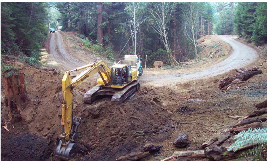
FIGURE 266B. Once cleared, an excavator excavated the fill material and several dump trucks were used to end-haul spoil material to a nearby, stable disposal site.
