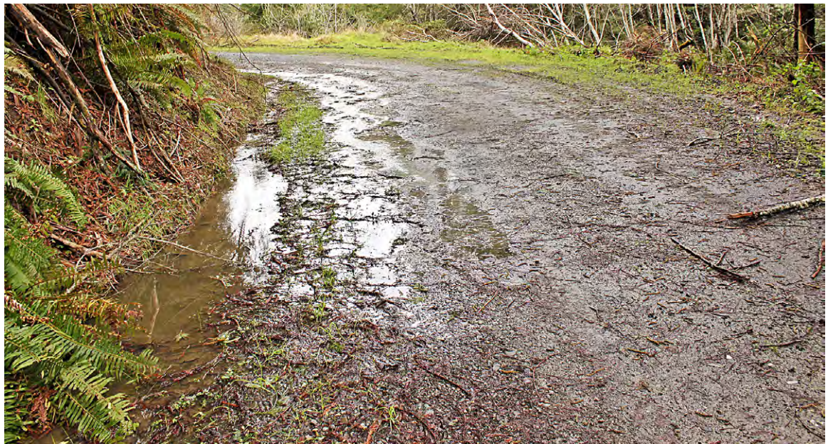
FIGURE 245. Over time, the ditch on this insloped road has filled with sediment. Road surface runoff now runs out of the ditch and onto the road surface, causing saturation and weakening of the road's structural section. Maintenance grading or excavation is needed to reestablish and deepen the ditch, thereby removing water from the road surface, draining moisture from the road base and surface materials, and re-strengthening the roadbed.
