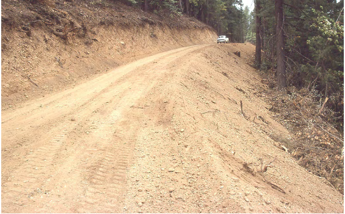
FIGURE 24. In contrast to the road in Figure 23, this partial bench road was built by extensive side-casting. At least half the roadbed is built on fill materials.
