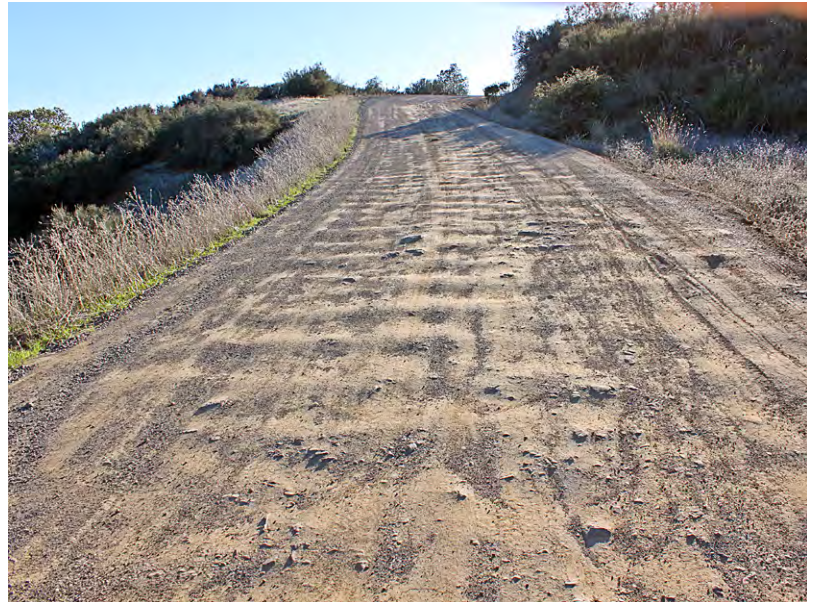
FIGURE 243. Steep road section where the road surfacing has broken down and moved off the road (maybe into a nearby stream), leaving behind the coarse base materials sticking up through the surface and making for slow traffic and a rough ride. This road needs scarification and the application of a new layer of road surfacing materials.
