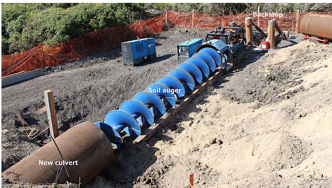
FIGURE 221. Tunneling is sometimes used to install a culvert in a deep road fill without opening an excavation or disrupting traffic. The large, powered soil auger drills and removes soil materials and fill from the hole and the new steel pipe is hydraulically jacked into the hole.
