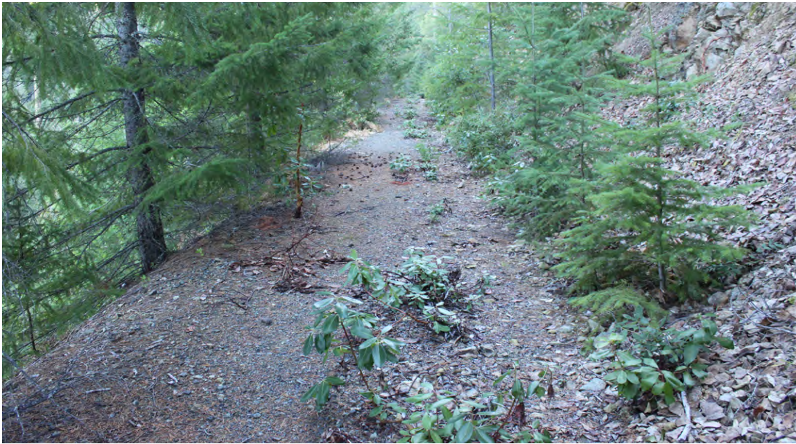
FIGURE 260. Untreated, abandoned section of forest road does not threaten water quality and needs little or no treatment for decommissioning. Roads to be decommissioned typically require minimal treatment for most of their lengths, and then concentrated erosion prevention work at a relatively few locations (e.g., stream crossings).
