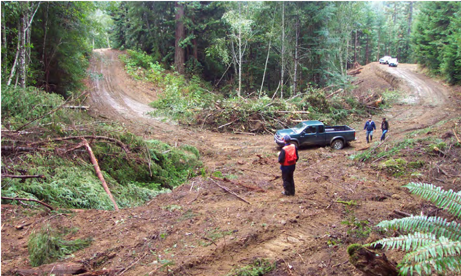
FIGURES 266A–E. This five-photo sequence shows the permanent decommissioning of a stream crossing on a former logging road. The road was no longer needed and has been permanently closed. The first step (266a) was to clear vegetation from the fill and from upstream of the crossing, where the channel had been filled with logging debris several decades earlier.
