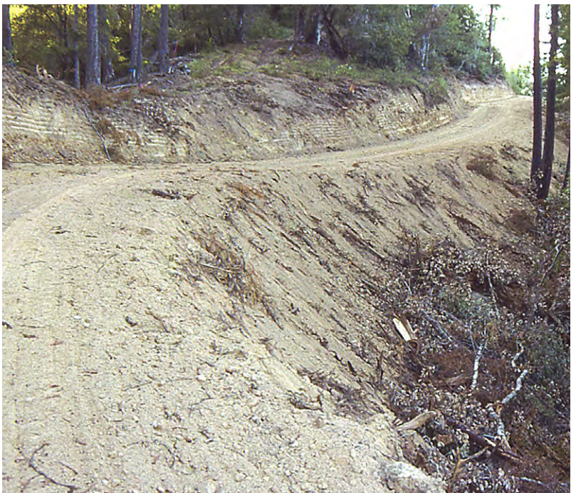
FIGURE 130. Road constructed by cutting and sidecasting (cut-and-fill road) in an upper hillslope location. A row of slash and organic debris along the base of the sidecast slope can help catch and filter soil eroded from the loose fill slope. Soil should only be sidecast onto gentle or moderate slopes that have been cleared and grubbed of vegetation, and where material cannot be eroded and delivered to a stream.
