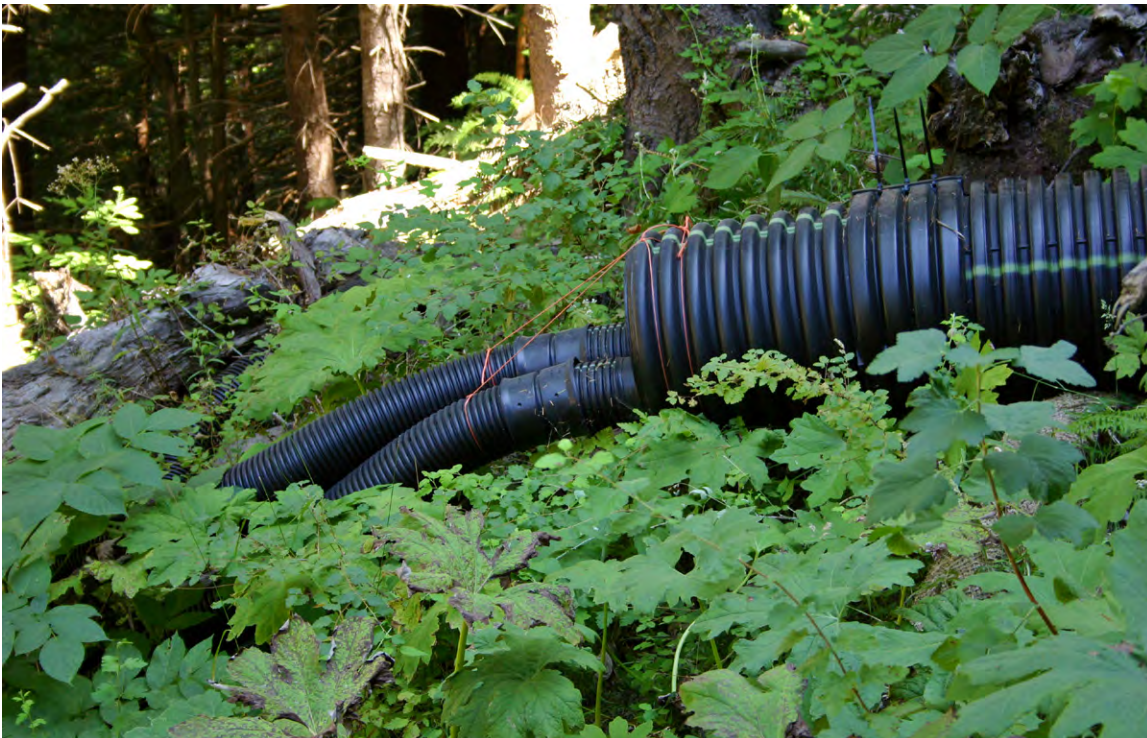
FIGURE 160. Ditch relief culverts on riparian roads that are very close to a stream channel are difficult to hydrologically disconnect. Here, an end cap and twin perforated flex pipes have been attached to the outlet of a ditch relief culvert. The perforated flex pipe is then staked along the slope's contour so turbid ditch runoff is slowly released and broadly dispersed along its length.
