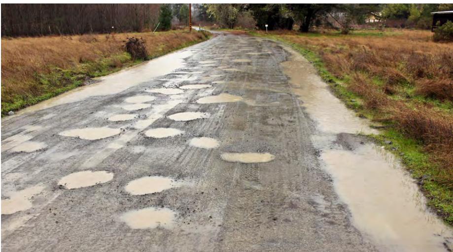
FIGURE 240. Slightly through cut, flat road exhibiting poor road drainage. Flat roads, with no gradient along or across the road, do not drain effectively and will develop potholes and mud puddles from continued traffic. Vehicles passing through standing water splashes the water and fine sediment from each hole or depression, gradually enlarging their size and depth. The through cut on this road developed by annual maintenance grading and the consequent gradual lowering of the road surface. Poor surface drainage will not improve until the road is raised and crowned, or paved.
