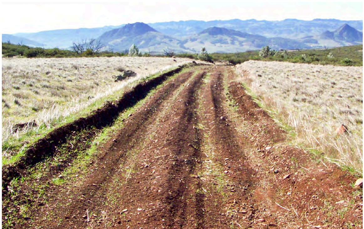
FIGURE 169. Road ruts on this seasonal road indicate a deteriorating subgrade that will either require traffic to be excluded during all but the driest periods, or strengthening with the application of a geotextile, base course, and surfacing materials.
