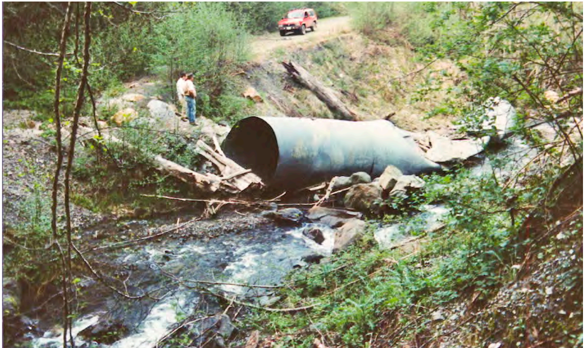
FIGURE 205. Under-designed or unmaintained stream crossings on older roads are prone to failure during large storms. This 8 foot diameter culvert was partially plugged (note wood at entrance) and flood flows overtopped and washed out the fill. During road reconstruction, stream crossings should be redesigned as temporary (and then removed) or upgraded for the 100-year flood flow, including passage of debris and sediment loads. When reconstructed, this crossing would either be fitted with an upstream debris screen or debris deflector, or a bridge would be installed.
