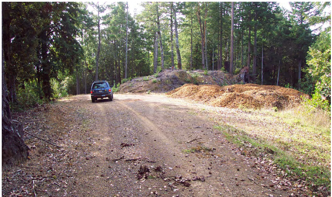
FIGURE 141. Typical spoil disposal site for endhauled spoil materials from a full bench road construction site. Spoil disposal site is located on a broad, gently sloping, dry ridge. Material is dumped, and will later be spread, compacted (by bulldozer) and seeded, mulched, and planted. Spoil material should be placed where eroded soil will not contaminate the road or ditch, or be delivered to a stream.
