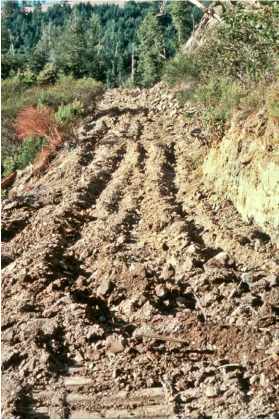
FIGURE 284. Deep, thorough ripping is a good treatment to largely eliminate surface runoff and “hydrologically disconnect” a former road from nearby stream channels.
