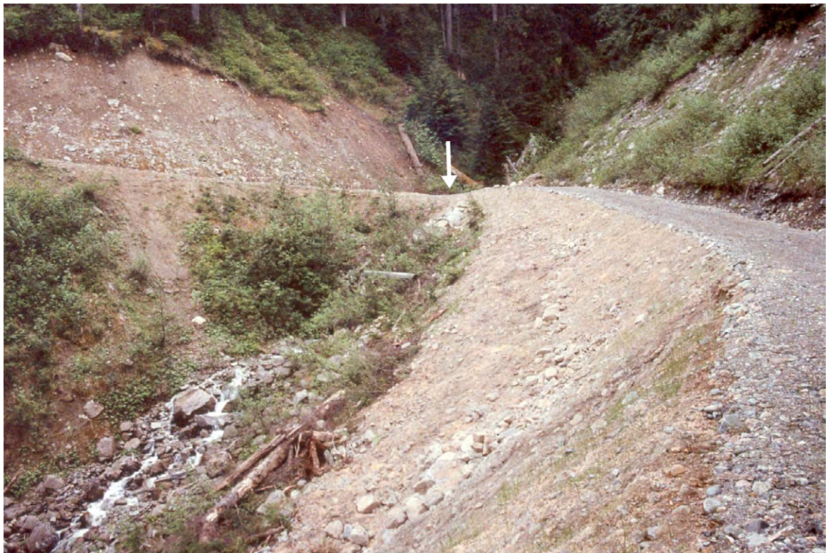
FIGURE 83. Critical dip at a stream crossing. Note reverse grade that directs flow over the road and back into the natural channel in this climbing road grade. Prior to installation of the critical dip, the culvert plugged and the stream diverted down the road and completely washed out the road in the foreground.
