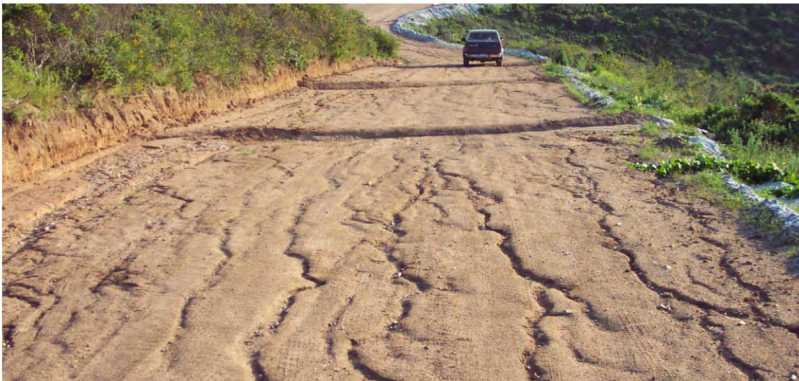
FIGURE 176. Road surface rilling on a steep seasonal road built on fine grained, erodible, native soils. Waterbars have been constructed to drain road surface runoff, but erosion occurs over even short sections of the exposed road.
