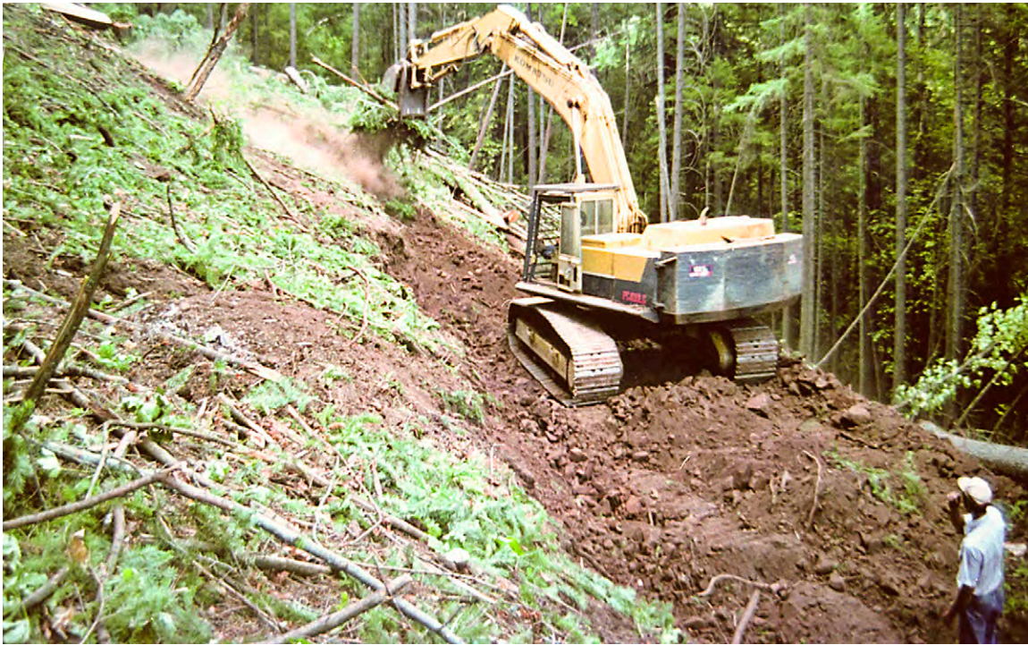
FIGURE 129. Hydraulic excavators have become the preferred piece of heavy earthmoving equipment for wildland road construction. Here an excavator is clearing and grubbing the alignment for a new forest road. All organic material must be removed from the alignment and woody debris should not be incorporated in fill materials.
