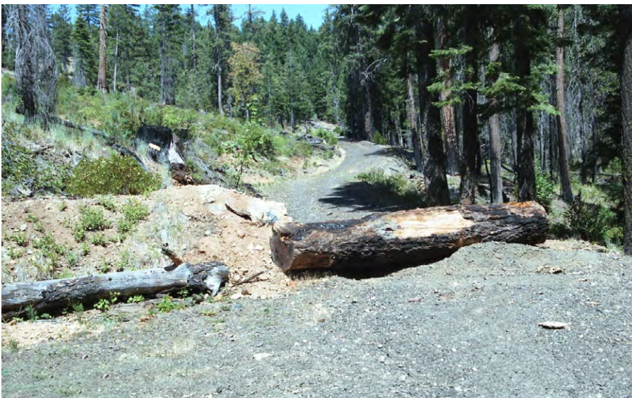
FIGURE 249B. If barricades or physical barriers are used, they must be removed with heavy equipment before maintenance activities can be performed. They should not be used on roads which have stream crossings since these need to be inspected and maintained during and following storms.
