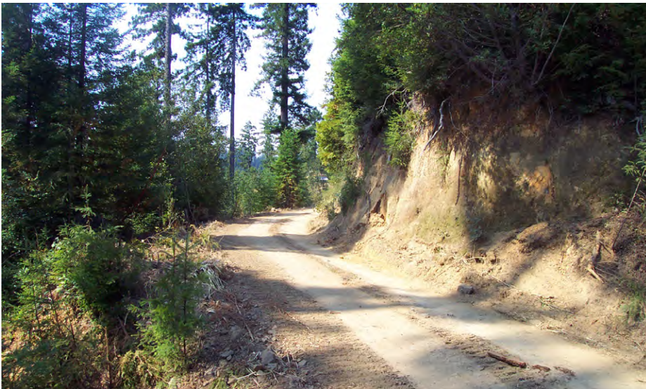
FIGURE 270A. Tall, dry cutbank where the road cut across the nose of a ridge. Just down the road an unstable fill was excavated to prevent a potential fill slope failure and this favorable site was used for spoil disposal.
