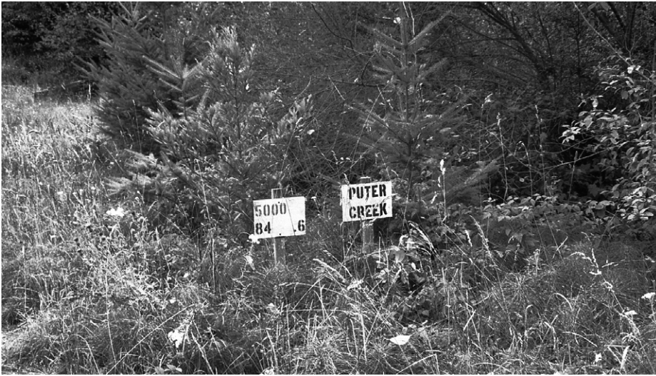
FIGURE 239. Culvert signing is an integral part of developing a culvert and drainage structure inspection and maintenance plan. Included at this crossing are the stream name (Puter Creek), the name of the road (5000 Road), the diameter of the culvert (84") and its location (0.6 miles from the beginning of the road). The signing can also be color coded (e.g., green, yellow, red) to indicate whether or not it is prone to plugging or other maintenance needs.
