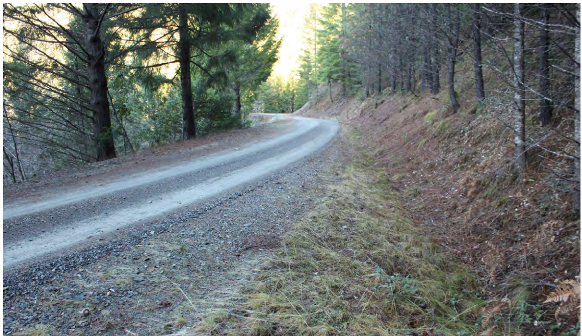
FIGURE 44. This insloped, gravel surfaced road drains to a vegetated ditch. The ditch is connected to a stream crossing culvert, but the heavy vegetation in the ditch prevents sediment from being delivered to the stream.
