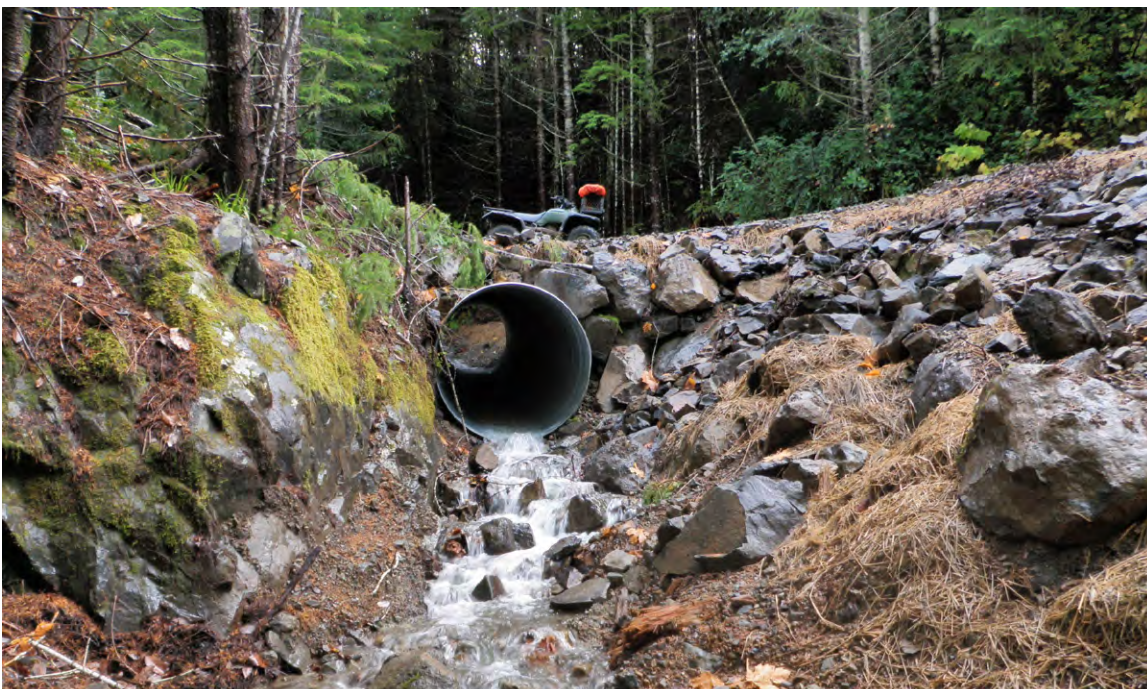
FIGURE 217B. The same stream crossing after culvert upgrading. The culvert has been set in the original streambed and the fill dipped to prevent stream diversion.
