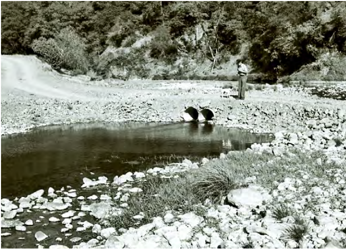
FIGURE 127A. Summer low-water crossing of a Class I (fish bearing) perennial river. Coarse, clean streambed material has been used to ramp up and over the flowing water. Two embedded culverts have been installed at water level to allow for uninterrupted flow and the migration of young fish.
