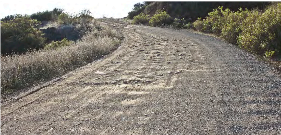
FIGURE 166. Road surfacing on this steep road reach has worn down the coarse base materials, making for a rough ride and reduced traction.
