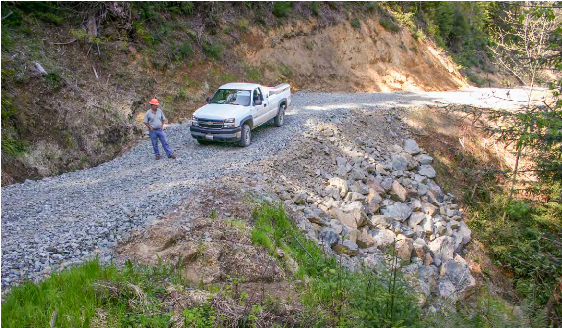
FIGURE 77. Road crossings of steep stream channels require fill slopes that often exceed a 2:1 slope gradient. This steep fill slope was stabilized with coarse rock armor embedded in a basal keyway.
