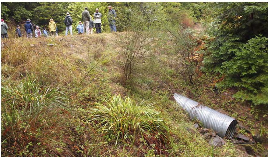
FIGURE 76. This newly upgraded 36-inch diameter culvert was installed in-line with the natural channel and at the base of the road fill. The road fill was graded to slightly less than 2:1 (50% slope) that was easily and rapidly revegetated. The culvert outlet extends at least 6 feet beyond the fill and discharges into the natural channel bed.
