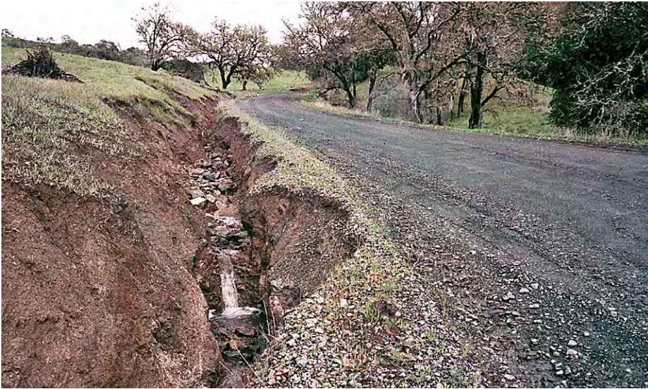
FIGURE 246A. Scoured roadside ditch carried runoff from the adjacent hillslope and from long lengths of the insloped road. The ditch gullied down to hard bedrock and discharged its runoff and eroded sediment to a stream just down the road.
