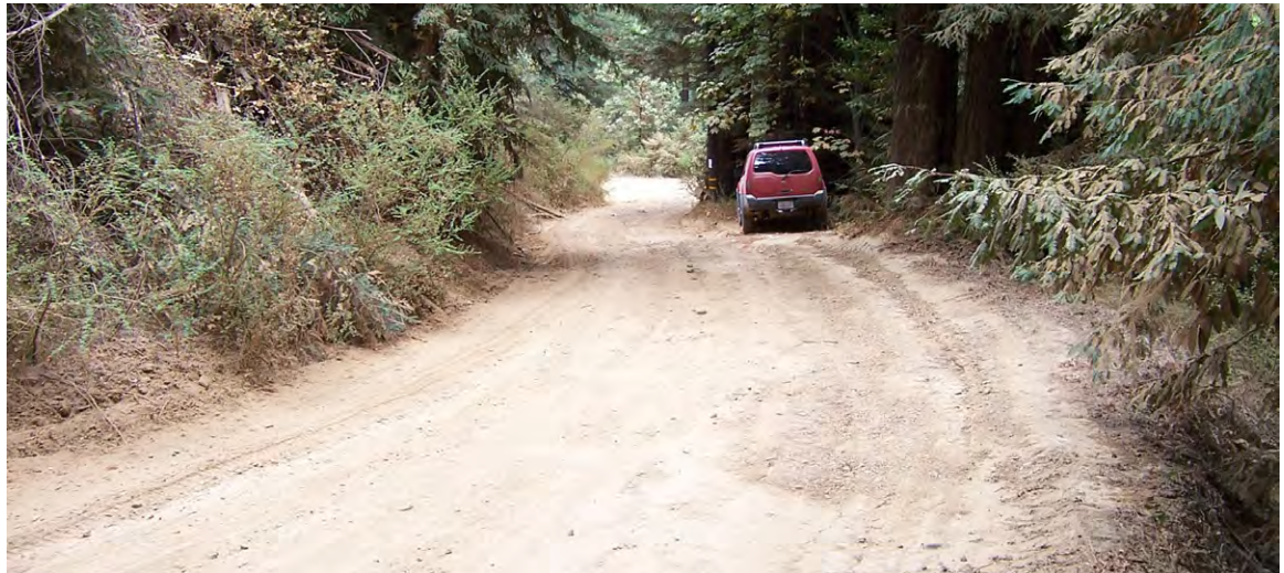
FIGURE 225A. Native surface permanent road on a rural subdivision was insloped, bermed, deeply rutted prior to upgrading and hydrologically connected to a nearby stream.
