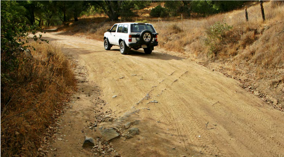
FIGURE 235. This road surface has worn down over years of use, grading and erosion to the point that a formerly buried ditch relief culvert has been exposed in the roadbed. When installed, the culvert was probably 2 or 3 feet below the road surface. Both gravel surfaced and unsurfaced (native) roads wear down over time, due to traffic and erosion. It is often not noticeable until the gravel is gone, the road becomes entrenched (through cut) or the top of cross drain culverts become exposed.
