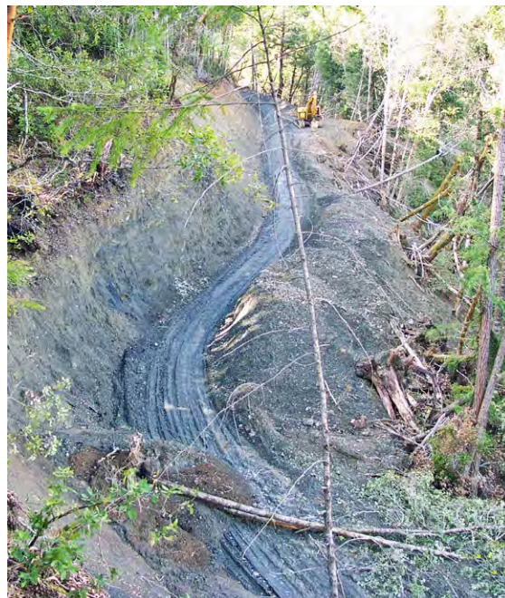
FIGURE 203. Sidecast constructed road built on a very steep inner gorge slope where a road should not have been built. Bulldozer constructed road perched large volumes of erodible spoil on the slope and debris slides have already delivered landslide debris to the stream channel below. This road is poorly located and upgrading will not reduce the failure potential. It is scheduled for permanent closure and the excavator (top of photo) is ready to begin decommissioning work.
