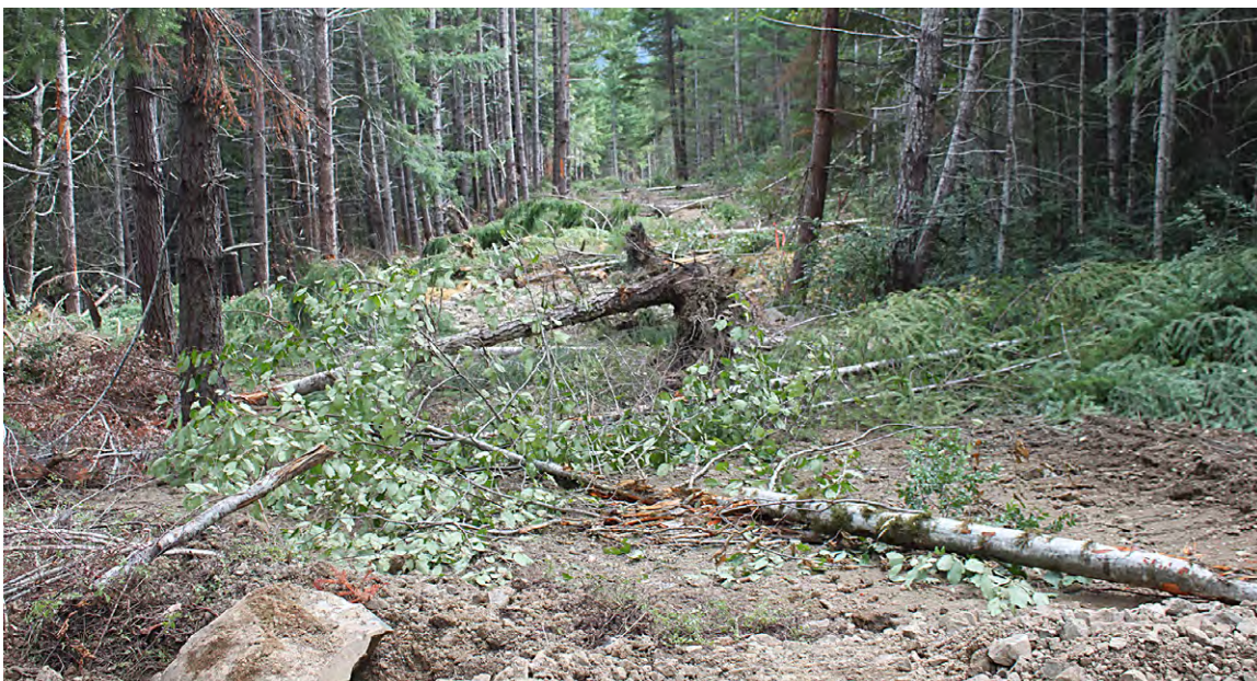
FIGURE 261. Decommissioned forest road in an area of gentle slopes and no stream crossings. Road decommissioning in “easy” terrain can be an inexpensive process that returns the former, compacted roadbed to productive forest or grasslands. Road decommissioning can be either permanent (never to be reopened) or temporary. The two treatments are generally similar and provide protection to the watershed for as long as the road is closed.
