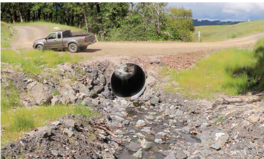
FIGURE 157B. After the first wet season (Figure 157b) the channel bed has self-armored and established a stable cross section leading to the inlet. Bare soil areas are covered with grass.
