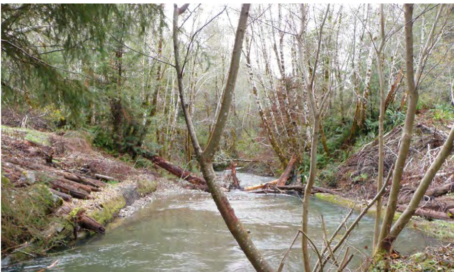
FIGURE 268B. Because the road was to be permanently closed, the bridge was removed as a part of road decommissioning. The lower, partially embedded abutment log on each side of the crossing was left in place to protect the newly excavated streambanks. The sideslopes were excavated and sloped back at a gentle angle, and then mulched with woody debris. Natural channel width was retained through the crossing.
