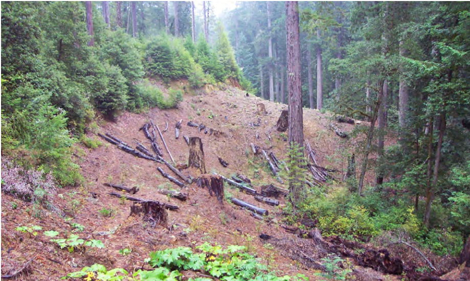
FIGURE 272B. After treatment, remnant stumps that had been buried by road construction and sidesteading were exhumed and gave the excavator operator a good idea where the original ground surface had been located. The outsloping was performed with little or no endhauling, as fill materials from the outside of the road prism were excavated, placed and compacted against the dry cutbank. Most of the cutbank has been buried and the slopes recontoured to their original form. The exposed soil was not seeded with grass, and rice straw was used as a mulch to prevent the introduction of non-native weeds. Litter from the adjacent forest quickly covered the surface.
