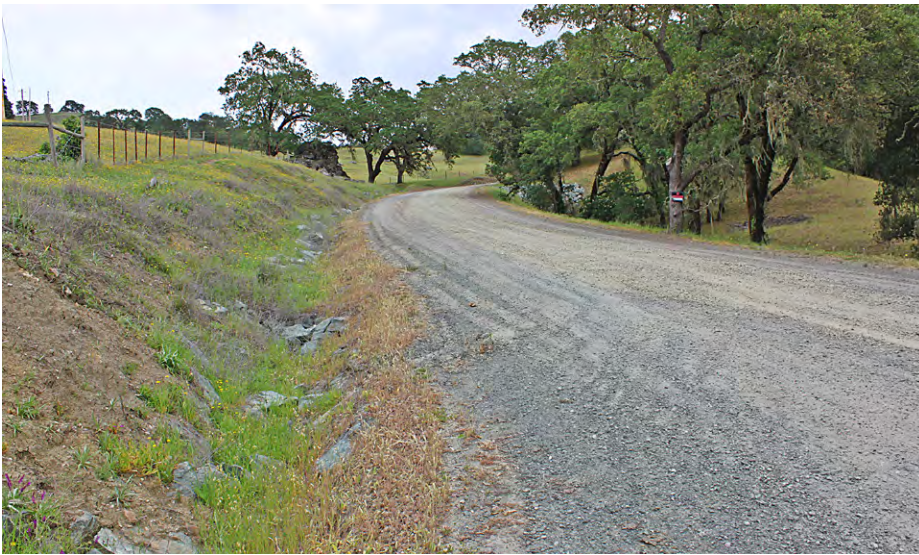
FIGURE 246B. The road was upgraded by crowning and additional ditch relief culverts were installed to disperse ditch flow. The pasture was also fenced to keep cattle off the erodible sideslopes.
