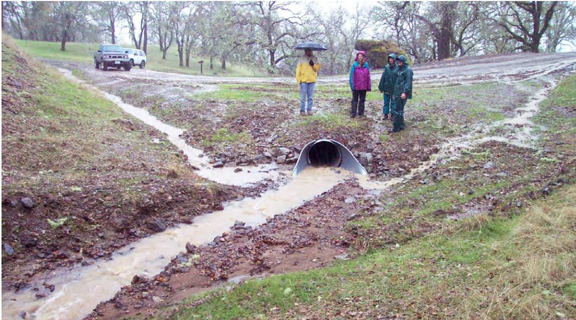
FIGURE 5. Hydrologic connectivity occurs where road and ditch runoff is delivered to the natural stream channel system. It most commonly occurs where road ditches discharge road runoff and eroded sediment directly to stream crossing culvert inlets. In this photo, both road ditches are hydrologically connected to the natural stream where it enters the culvert.
