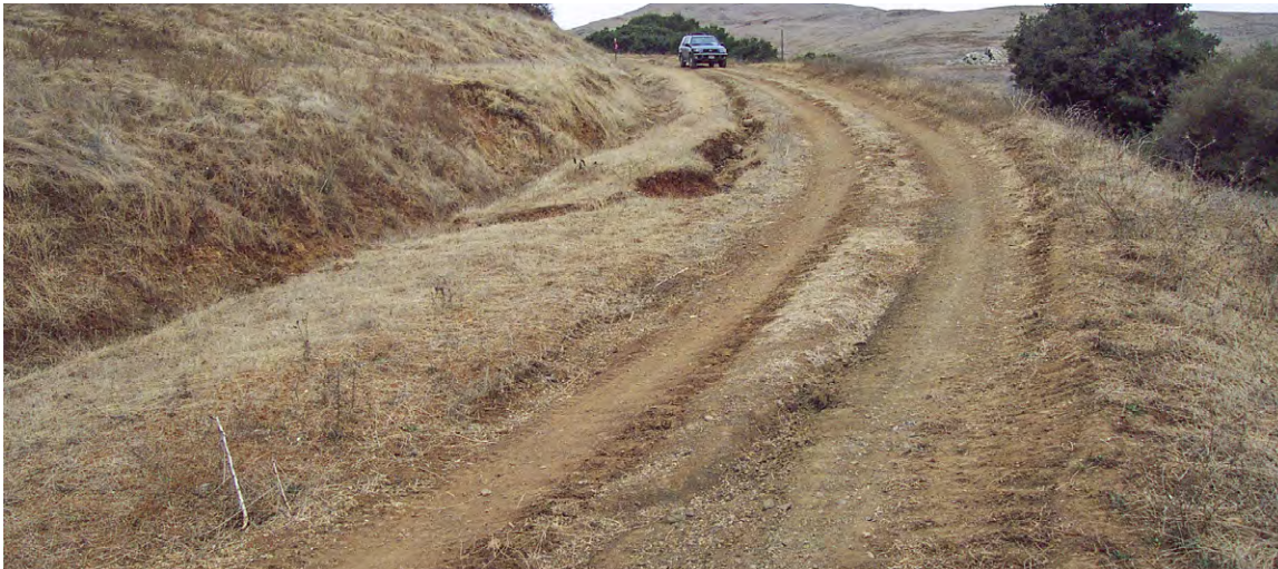
FIGURE 224A. Ditched, gullied, deeply rutted, and bermed seasonal road before being converted to an outsloped road with rolling dips.
