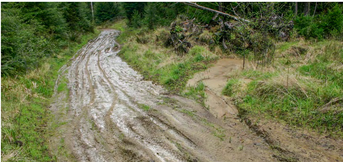
FIGURE 57. This seasonal road was built on fine grained soils that exhibited poor drainage and high rates of soil erosion. Even minor traffic during the wet season caused damage to the roadbed and rapid erosion clogged and filled ditches, waterbars and rolling dips.
