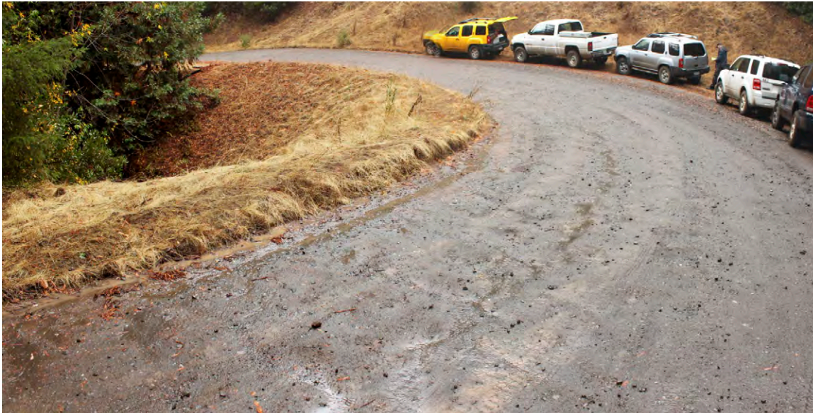
FIGURE 82. This newly upgraded stream crossing fill was protected from road runoff and erosion by the installation of a drainage berm along the road. Once the fill is vegetated and stabilized, the berm can be safely removed.
