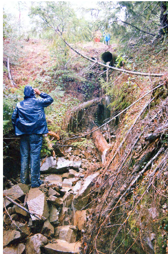
FIGURE 201. A road inventory crew surveys stream crossings and other under-designed elements of a road, identifying needed upgrades along the route. The most important things to identify, and upgrade, are those that could cause road or stream crossing failures (like this perched, undersized stream crossing culvert), or that deliver road runoff and fine sediment to the stream system.
