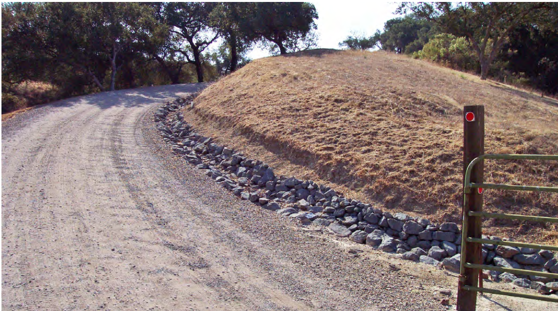
FIGURE 184. Rock armored ditches, if constructed with proper rock sizes, rock gradations and U-shaped channel form, can prevent ditch downcutting and erosion, but also inhibits easy ditch maintenance using machinery. Rather than armoring or installing check dams in ditches, it is usually best to reduce the volume of flow by installing additional ditch relief culverts.
