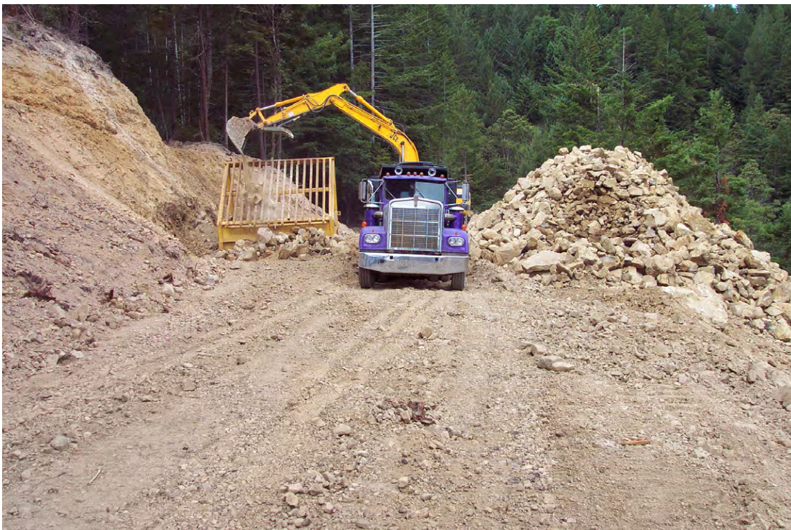
FIGURE 60. This rock pit is easily worked by an excavator, but the material contains abundant fine grained particles. Here, a Grizzly rock screen is used to separate high quality rock armor from fine grained waste materials. As in this photo, waste materials should be endhauled to a stable spoil disposal site rather than sidecasting onto steep, unstable or streamside slopes.
