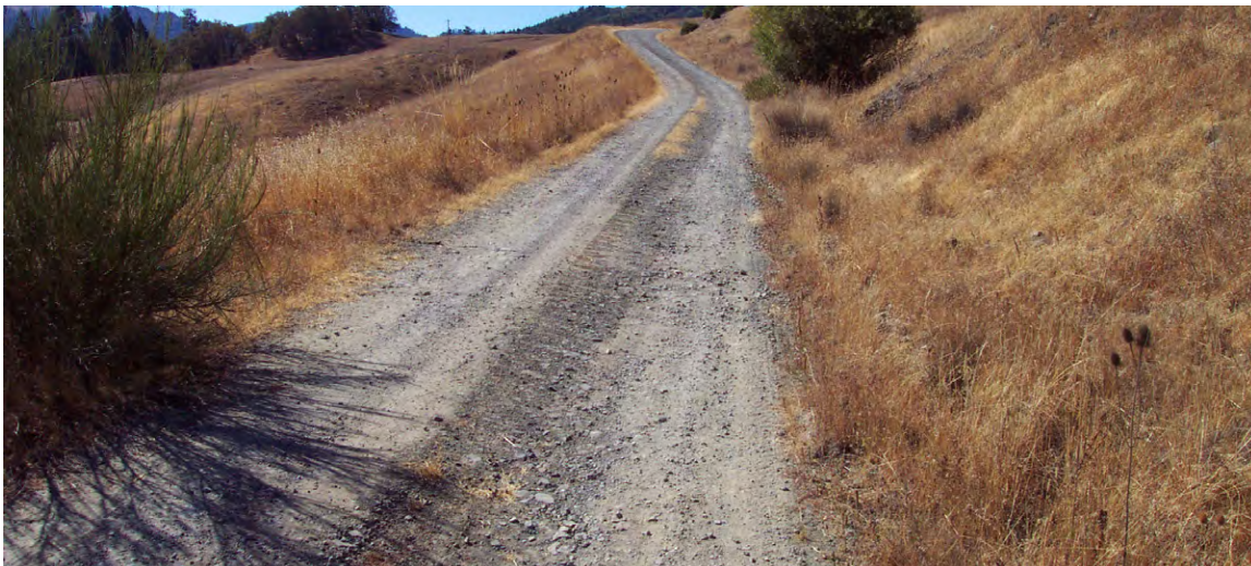
FIGURE 226A. Rural subdivision road was insloped and rutted prior to treatment. Runoff from the eroding roadbed was delivered directly to a stream channel.
