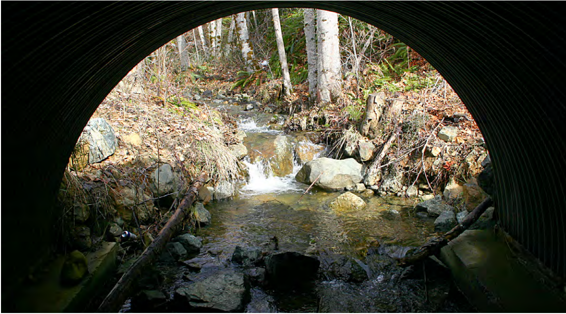
FIGURE 233. View looking upstream through the inlet of a newly installed bottomless arch. The stable boulder bed of this stream ensures the foundations will not be undermined by channel downcutting. For flow capacity, and to prevent plugging with debris, the basal span of the arch has been built wider than the natural channel.
