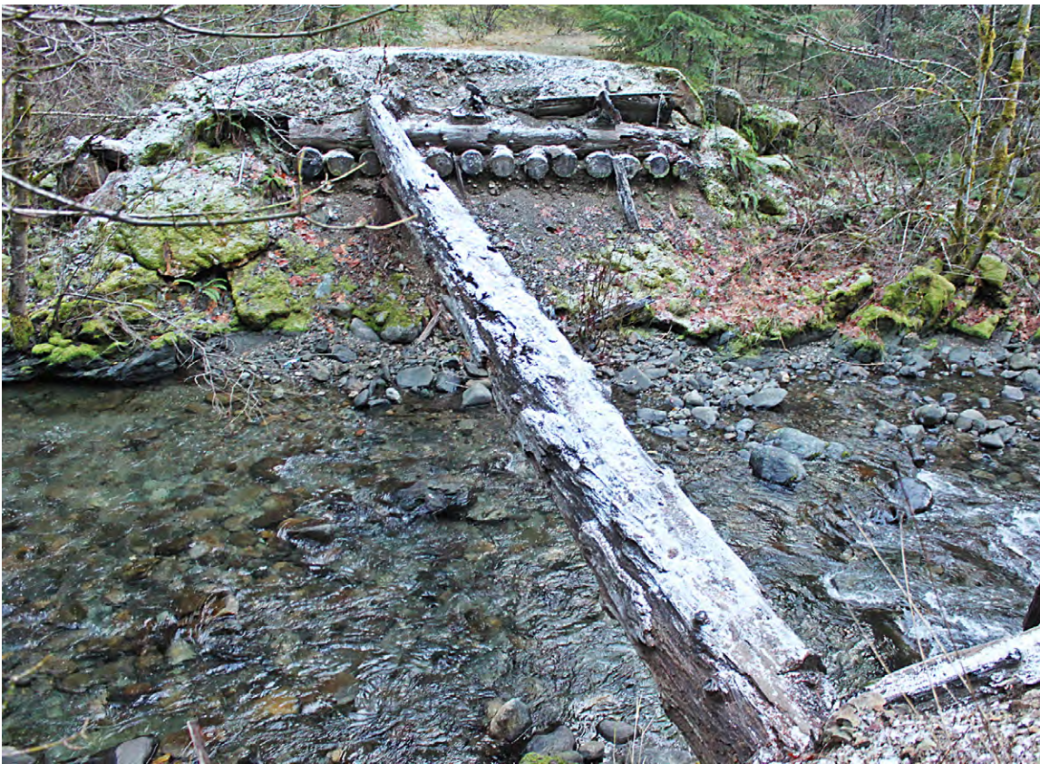
FIGURE 257. Former log stringer bridge across a large fish bearing stream has been removed, with only a single log for left foot traffic. The bridge provided the only access to over two miles of forest road containing numerous culverted stream crossings that can no longer be maintained. Roads that have not been properly decommissioned require inspection and maintenance. The roads on the other side of this bridge have recently been scheduled for decommissioning.
