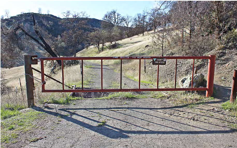
FIGURE 249A. There are a variety of ways to close a road to off-season traffic, but it should always be remembered that barricading the road does not by itself prevent erosion along the alignment. Gating closes the road to unauthorized traffic but still allows for winter maintenance and inspections.
