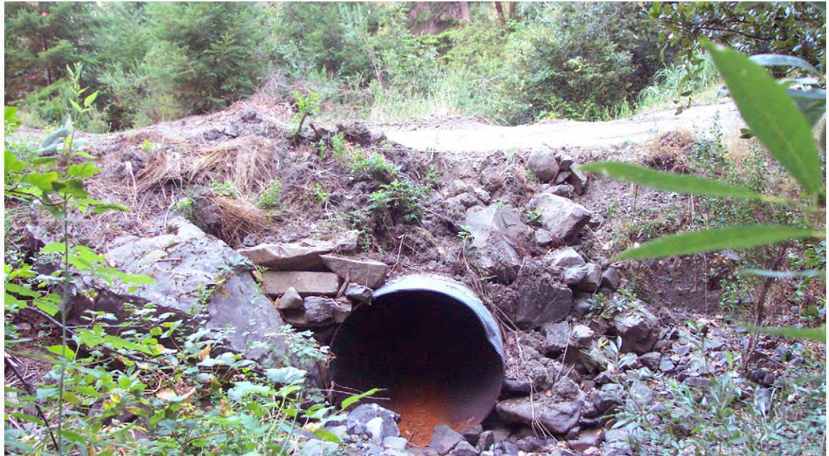
FIGURE 232A. This 48-inch diameter culvert is significantly undersized for the design flow event. The culvert inlet has plugged during past storm events and flood flows were diverted down the road, creating a large hillslope gully.
