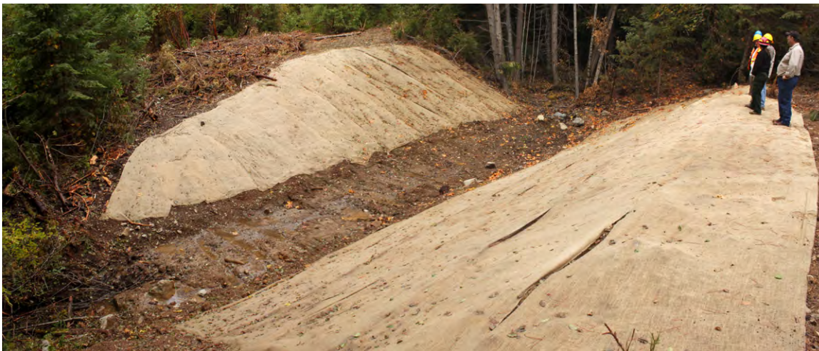
FIGURE 281. Most often, a uniform cover of straw mulch is all that is needed to temporarily control surface erosion on the excavated sideslopes of decommissioned stream crossings until they can naturally revegetate. Wood chips, or native brush and slash, also work well to control surface erosion in some environments. Here, jute netting has been used instead of straw, as a trial treatment. Rolled and tacked erosion control blankets, or jute netting tacked over a layer of straw mulch, can be used on sideslopes that are steeper than about 2:1 (50%). To avoid spreading non-native weed species, many areas can employ rice straw whose seed and weed species are not adapted to growing in most upland environments. Rice straw mulch also has a roughness or “stickiness” that allows it to hold in place on slopes steeper than wheat or grass straw.
