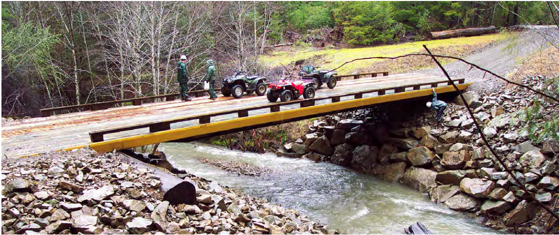
FIGURE 116. Low cost railroad flatcar bridges can be used for temporary crossings of incised stream channels, or they can serve as permanent water-course crossings. This 65-foot bridge spans the entire channel and was placed on large log abutments. The side-slopes have been protected with heavy rock riprap, and the natural channel width has been maintained through the crossing.
