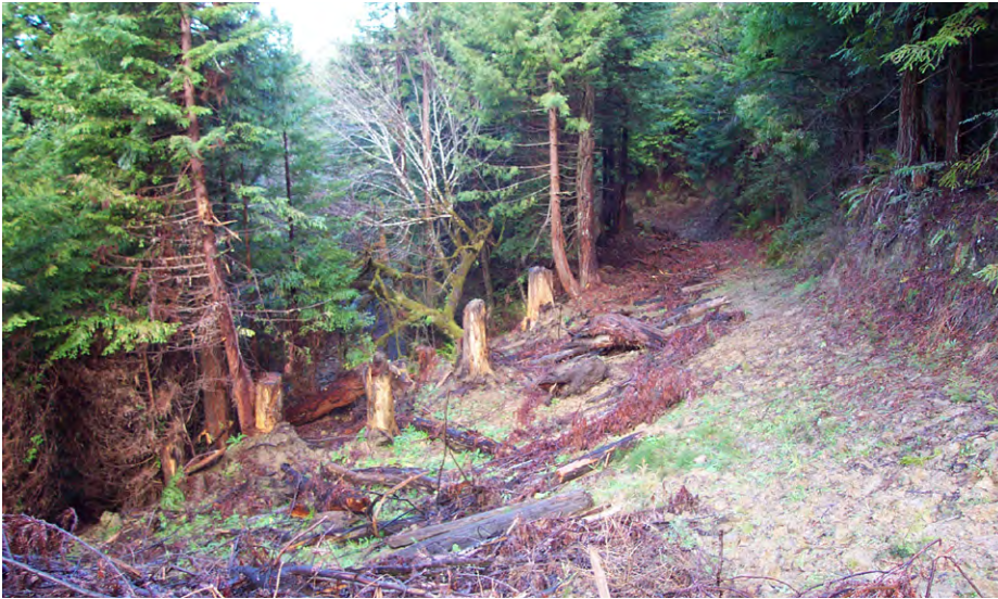
FIGURE 269C. The fill slope has been excavated and the spoil endhauled to a nearby spoil disposal site (exported outslope: EOS). Note the buried stumps that were exhumed and the basal flair that told the excavator operator where the original ground surface was located and how deep to dig. The cutbank has not been buried so the resulting outslope of the former road bench is strictly a result of roadbed and fill slope excavation.
