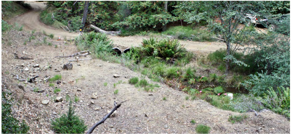
FIGURE 218A. Dual, undersized culverts were a partial barrier to fish migration on this rural road.
