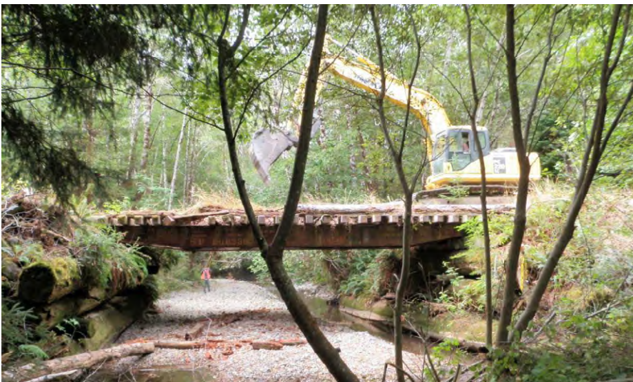
FIGURE 268A. Abandoned road and flatcar bridge over a large fish bearing stream. Unlike log stringer bridges, which are often covered with a thick layer of soil, flatcar bridges do not have a cap of soil that could enter the stream when they eventually fail. However, the log abutments were beginning to collapse and the collapsed logs and bridge would likely cause future flow deflections and channel erosion.
