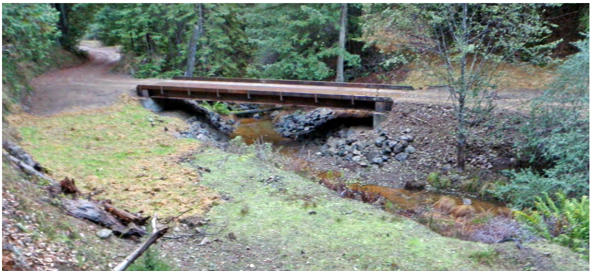
FIGURE 218B. The culverted stream crossing was upgraded to a flat car bridge to provide for passage of adult and juvenile fish. Note the concrete abutments, armored fill slope and naturally wide channel bottom through the crossing after bridge installation.
