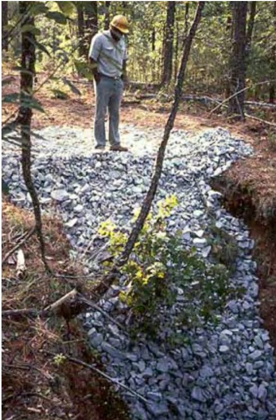
FIGURE 179. Rock mattress at gully head armor the headcut and conveys surface flow to the stable channel below (USDA NRCS, 2007).
