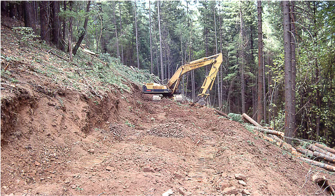
FIGURE 131. Excavators can perform a simple three step process of clearing and grubbing, excavating and subgrade development during construction of a balanced bench road. Using an excavator minimizes the volume of sidecast material. In the first pass an excavator operating from a pioneered bench removes logs and stumps, grubs the slope and installs a filter windrow of slash material at the base of the proposed fill slope. The second task is for the excavator to remove the overburden and place and compact the fill on the bench it has created (see piles of clean soil) and downslope above the windrowed slash. Thirdly, the uncovered, unweathered material is used to construct the bearing surface of the road.
