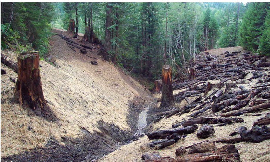
FIGURE 266C. The channel was excavated (exhumed), and the side-slopes were sloped back to stable angles, exposing several buried stumps that signaled the level of the original ground surface. The bare slopes were then seeded, mulched with straw, and planted with trees. All the logs visible on the right bank had been buried in the crossing fill. They were removed and placed on the final ground surface.
