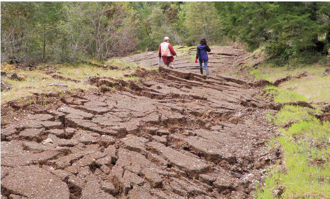
FIGURE 206. This rural road traversed a large unstable hillslope that showed widespread movement during an exceptionally wet winter. The road did not cause the instability but it is no longer useable. Alternative access should be developed wherever roads cross highly unstable terrain. This road should be decommissioned so no additional erosion and instability is caused by the road and its drainage structures.
