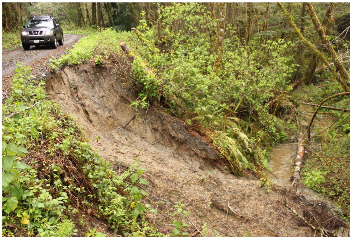
FIGURE 4B. At a smaller and more common scale, fill slope failures on roads built on steep slopes near stream channels have a high likelihood of delivering sediment directly to the stream channel.
