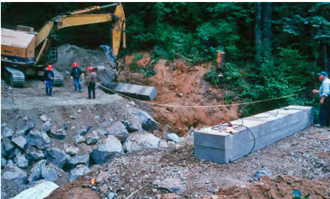
FIGURE 149. Bridge abutments can be built of logs, piers, concrete pads, and other supports. This abutment is a precast concrete support that was fabricated off-site and installed when road construction reached the crossing location. A level pad for each abutment is excavated, base material spread and compacted, and the prefabricated concrete abutments placed and measured for the specific bridge.
