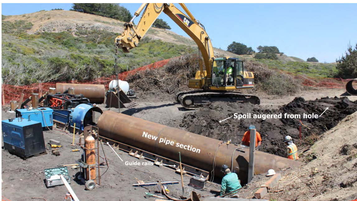
FIGURE 222. New pipe section is welded to the previous "jacked" section and the process is repeated until the outlet is exposed at the base of the outside fill slope. Guides along the ground are used to keep the pipe and auger aligned and straight. Soil removed by the auger is endhauded to a spoil disposal site.
