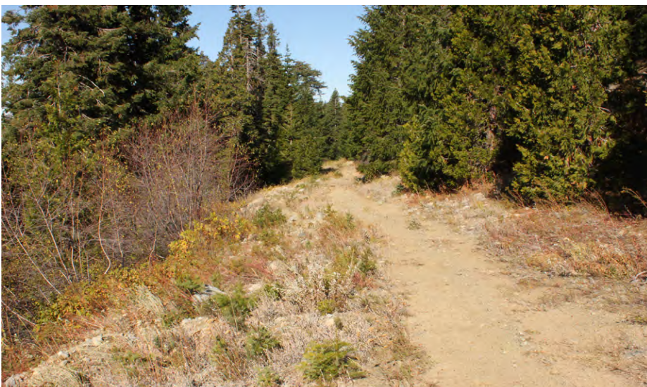
FIGURE 279. Former forest road that has been ripped, slightly outsloped and converted to a hiking trail. The decommissioning treatment needed in this upper hillslope setting was minor and yet largely eliminated surface runoff from the alignment.
