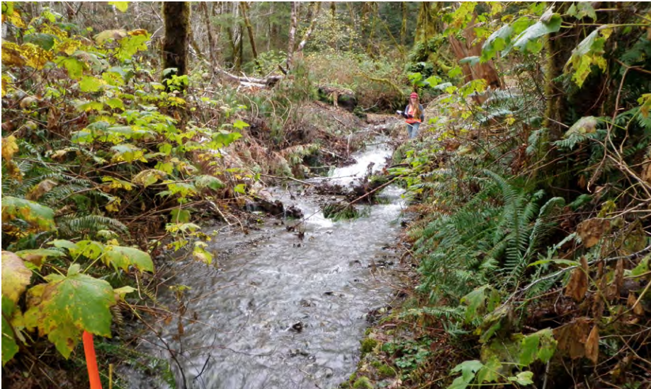
FIGURE 267B. The stream crossing fill was excavated and pushed down the alignment, away from the crossing. The gentle, excavated sideslopes were seeded, mulched with straw and covered with locally derived tree limbs and brush. The channel was excavated to the original streambed elevation, where rounded cobbles were exhumed, and constructed with the same width as the upstream and downstream channel reaches.
