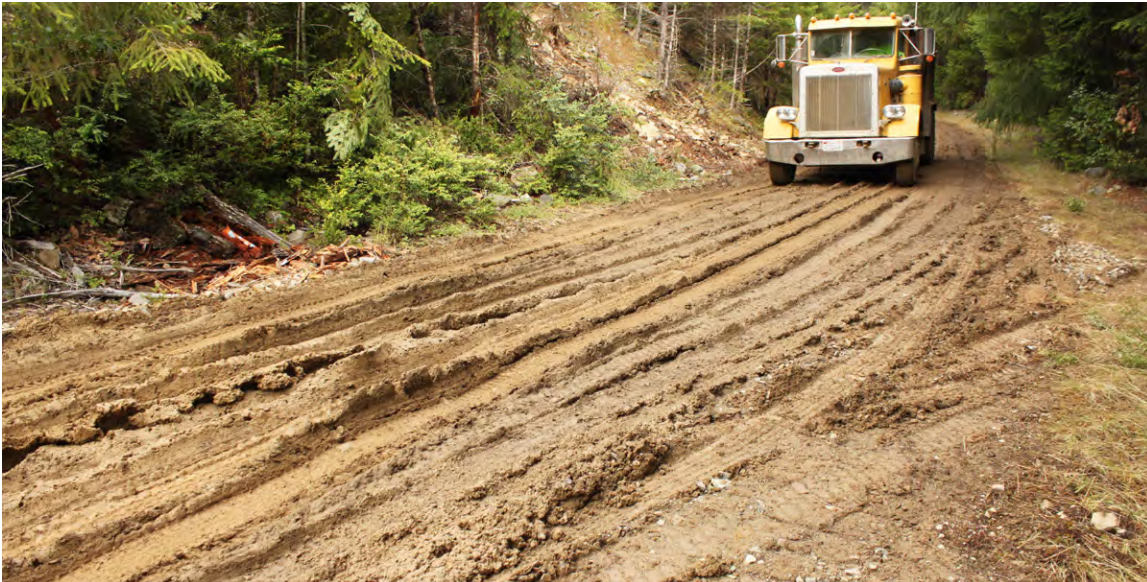
FIGURE 237. Roadbed structural deterioration caused by vehicle traffic (especially commercial traffic) on wet subgrade soils with little or no surfacing. Wet weather road use limitations (gating) or road surfacing (with base and surfacing materials) are preventive solutions to this potentially expensive maintenance problem.
