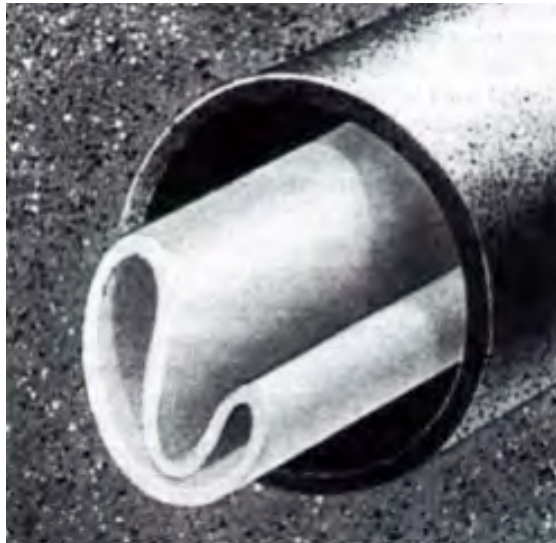
FIGURE 219. ‘Fold and form’ culvert liner.
