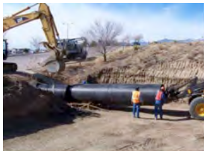
FIGURE 220. Sliplining technique for trenchless pipe installation.
