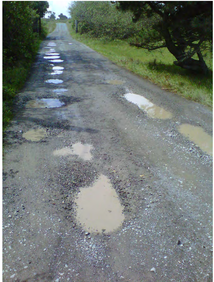
FIGURE 168. Standing water and the development of potholes are common indicators of poor road drainage.
