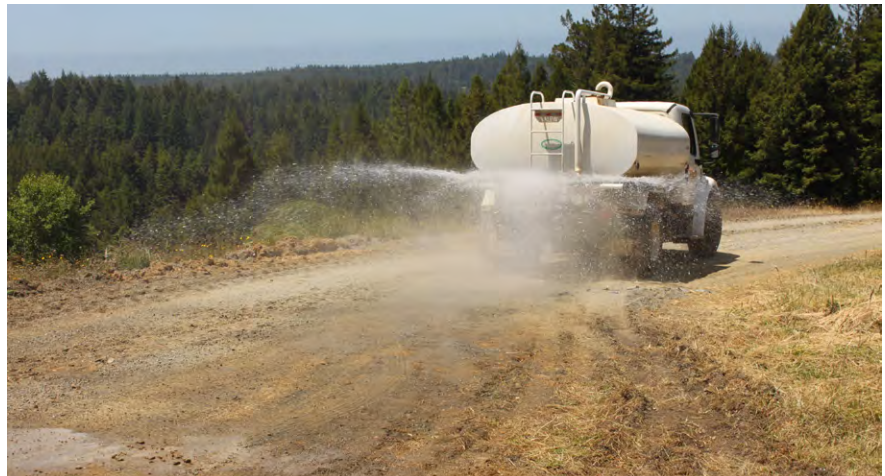
FIGURE 241. Water trucks can be used to apply water needed for compaction or dust control at project sites or along high traffic routes, or for applying a dust palliative (e.g., MgCl) for longer term dust control.
