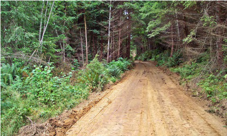
FIGURE 278A. On forest roads which are to be formally closed, rather than just “abandoned,” the roadbed can be returned to forest or grassland production by ripping and disaggregating the surface and then planting with trees. Figures 278a and 278b show a road before and after ripping and decompaction. This simple, inexpensive treatment also helps reduce runoff from compacted areas. It is recommended that enough passes be made with the tractor so the surface is completely disaggregated.
