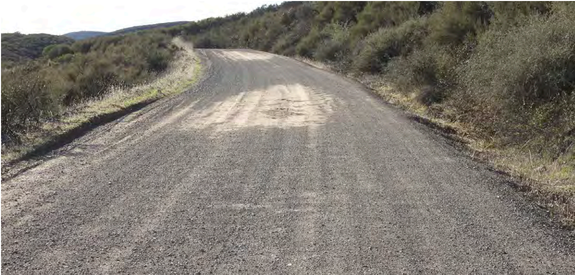
FIGURE 165. Because of traffic and erosion, road surfacing has locally worn down to the lighter color, finer grained native base materials beneath. The road needs resurfacing.
