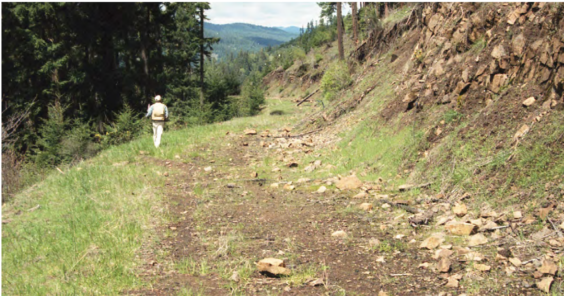
FIGURE 11. Seasonal roads are built to the same specifications as permanent roads, but are not surfaced for all-weather traffic. They typically provide summer or dry period access to watershed areas. The potentially erodible road surface may be waterbarred before each winter (not shown), or outsloped with rolling dips to provide for rapid drainage of surface runoff.
