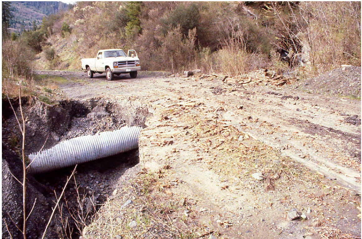
FIGURE 64. Eroding stream crossing after a single storm on an unmaintained road. The culvert plugged and flood flow overtopped the fill, initiating a head-cut. In addition to being undersized, the culvert was installed at a flat gradient that is more prone to inlet plugging with debris. If left uncorrected, the crossing fill would continue to erode and deliver the eroded sediment downstream.
