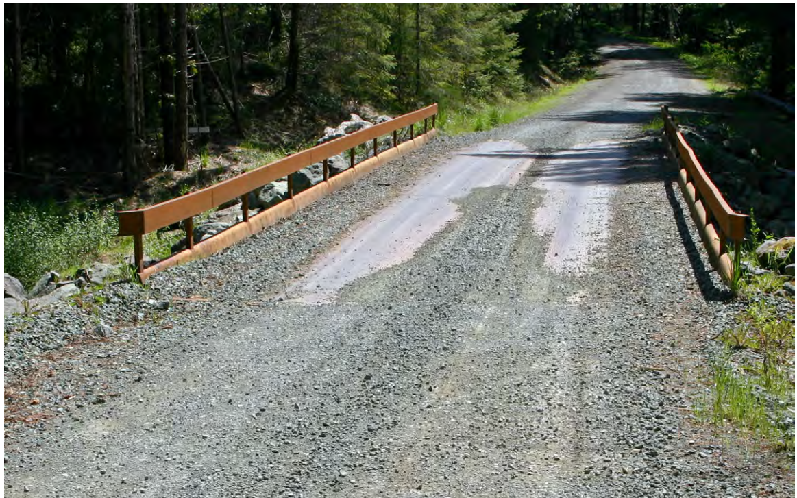
FIGURE 154. Wheel guards on a railroad flatcar bridge (see Figure 153) signal the driver that he is too close to the edge of the bridge. On this flatcar bridge, the road in the foreground slopes down to the bridge but the continuous steel wheel guard also seals the bridge surface so that all road runoff and sediment flows across the bridge and farther down the road before being dispersed onto the vegetated hillslope.
