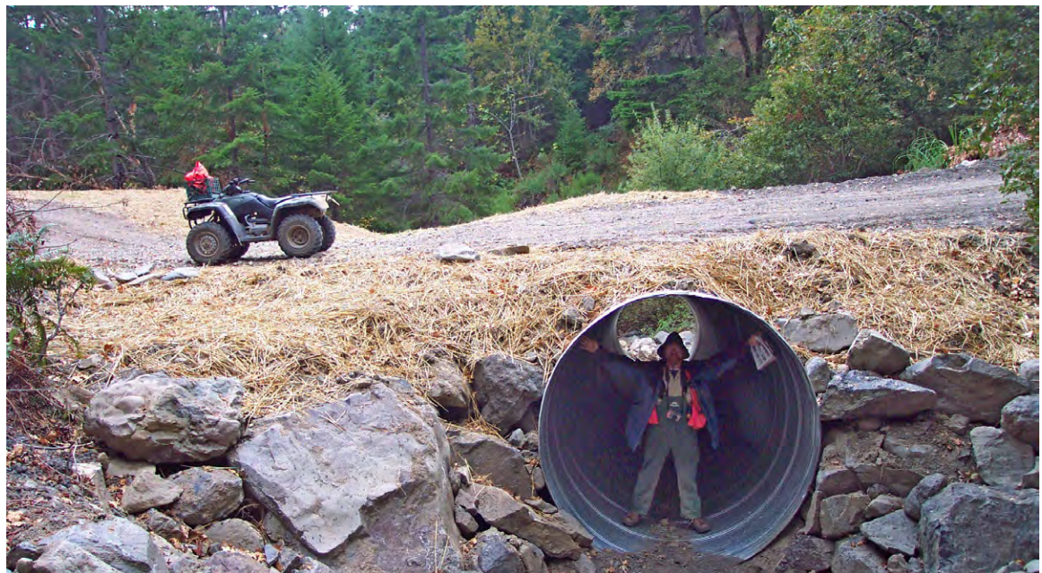
FIGURE 232B. The stream crossing was upgraded with an 84-inch diameter culvert, the inlet area was armored, and a critical dip was installed on the left hingeline of the fill to prevent future stream diversion if the culvert was to plug.
