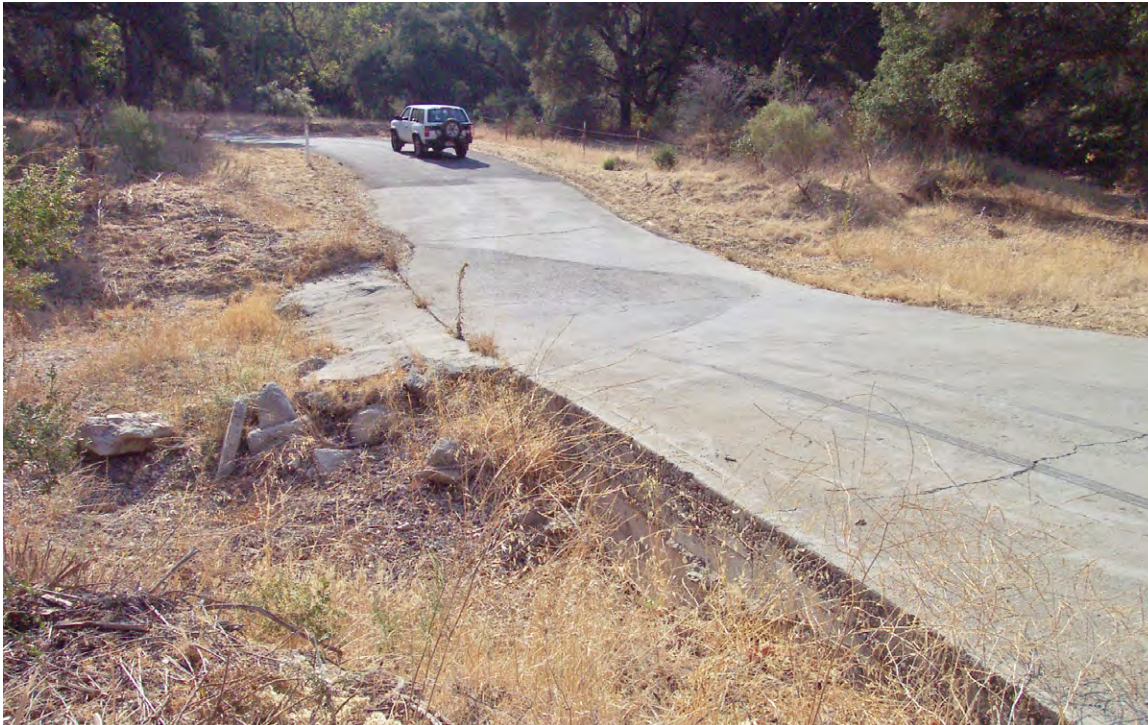
FIGURE 123. Flow in this hardened ford is from right to left. Low flow energy dissipation has been built into the center of the structure, but high flood flows have scoured to the base of the concrete ford in the foreground. Both the hardened ford and the downstream energy dissipation must be broad enough to encompass and contain the expected 100-year design flood flow.
