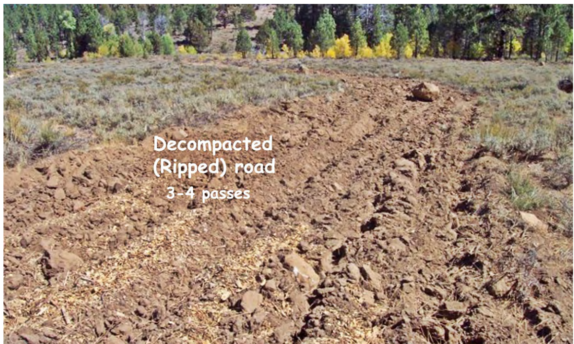
FIGURE 280. On gentle terrain, ripping (soil decompaction) maybe the only treatment that is needed to decommission a road, eliminate unwanted traffic, reduce runoff and return it to native vegetation.
