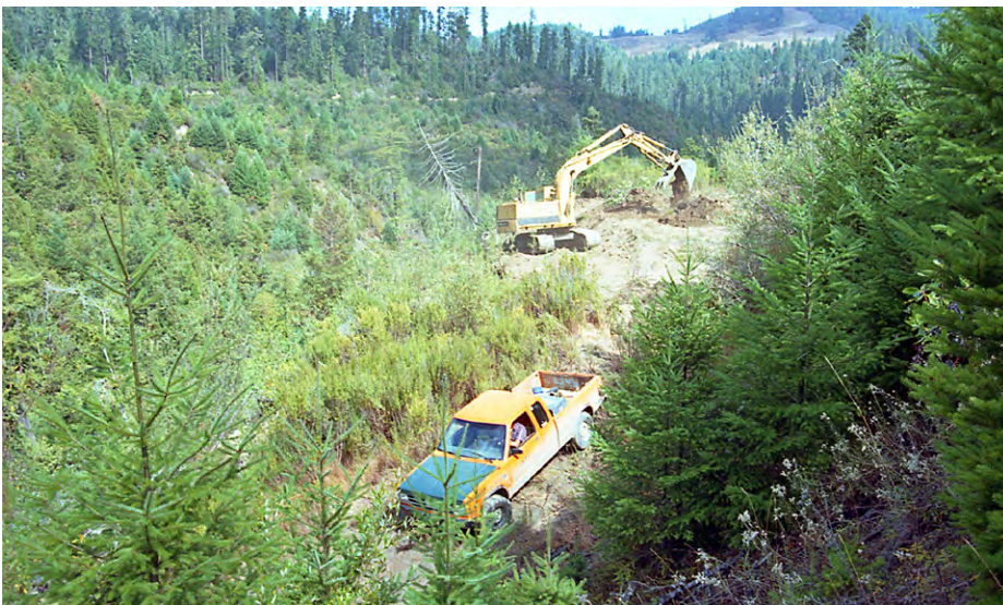
FIGURE 273A. Log landing on a forest spur road had developed large cracks and scarps around its outside perimeter where soil and wood waste had been sidesteamed onto steep slopes above a fish bearing stream. The fresh scarps had developed over several years and were identified by an inventory crew surveying for erosion problems in the watershed. An excavator is beginning the fill slope excavation and spoil material was pushed against the inside of the landing by a bulldozer (not visible).
