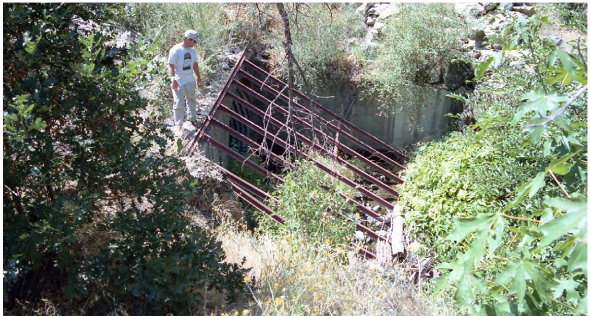
FIGURE 99. This 6-foot diameter culvert with concrete head- and wing-walls has a trash screen built over the inlet to catch floating debris. The design is flawed because it screens and catches small woody debris that would otherwise easily pass through the culvert. During a flood event, debris will quickly cover the trash screen and effectively plug the drainage structure. Screen bars should be more widely spaced and the trash rack should be installed in the stream channel somewhere upstream of the culvert inlet.
