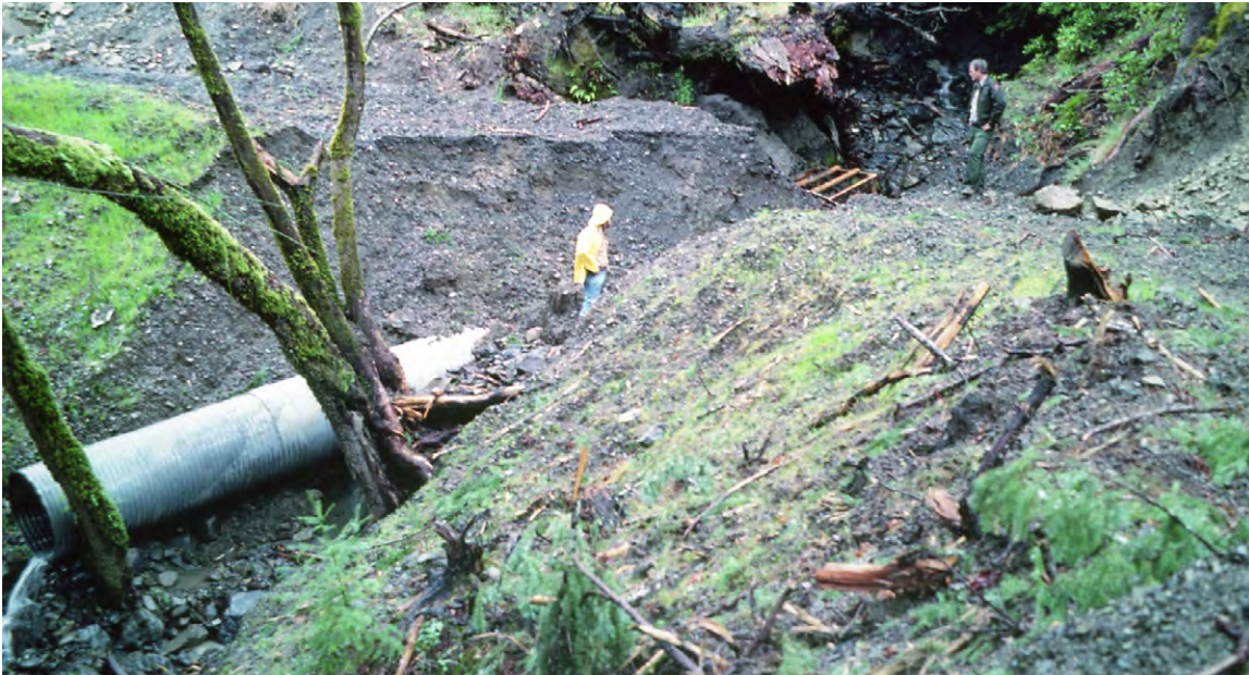
FIGURE 2. This stream crossing “washed out” (eroded) when the culvert plugged and streamflow overtopped and scoured through the road fill. Sediment was delivered directly to the stream system as the fill eroded. Stream crossings and culverts need to be properly designed, constructed and maintained to minimize the potential for such failures.
