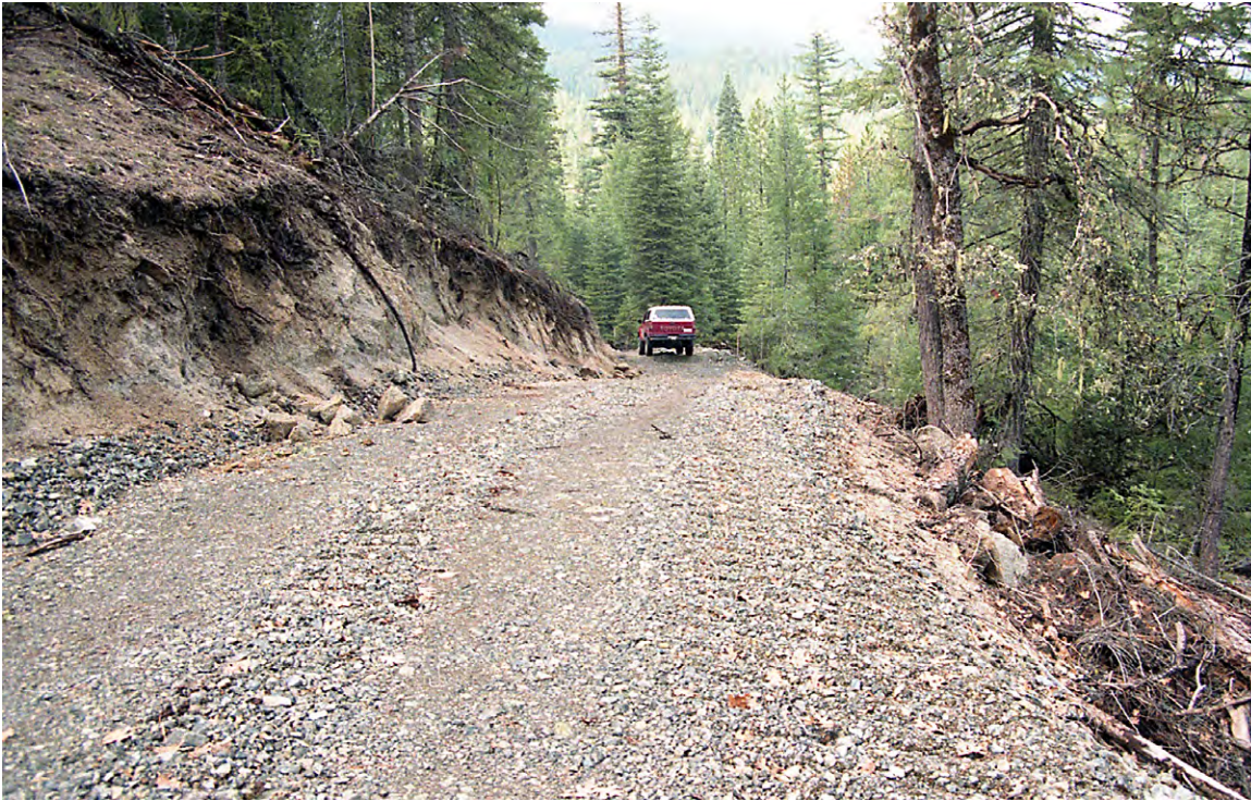
FIGURE 172. Newly constructed, outsloped forest road with accumulated line of slash, called a filter windrow, at the base of the fill to catch soil eroded from the new fill slope. Slash should be placed at the base of the fill, and not incorporated into the soil material. Filter windrows are most important to install where roads approach and cross stream channels. This outsloped road conforms to the topography of the land and incorporates rolling dips at natural swales to shed surface runoff.
