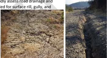
Figure 6: Rills on a road surface (left) and a gully formed on a road surface (right)
