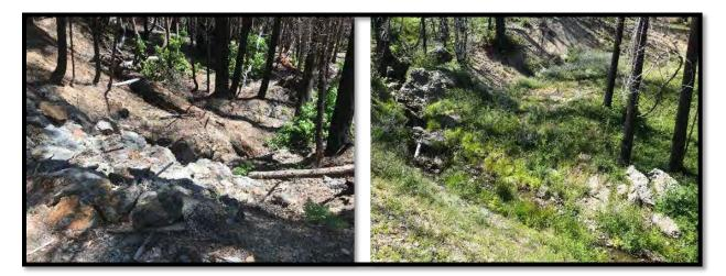
Figure 54. Armored crossing drainage on a Class III in the Cascade area, left, in a post fire Emergency Notice, that was recorded as having a trace amount of sediment discharge. An abandoned crossing on a Class II post-fire Emergency in the Cascade Region, right, that resulted in less than one yd<sup>3</sup> of sediment discharge based on field observations
