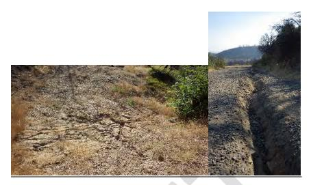
Figure 4: A road surface with rills (Left) and a gully formed (Right).
