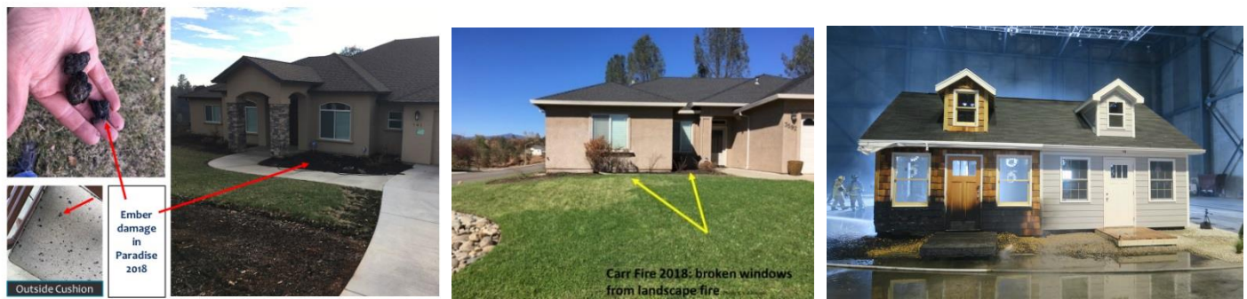
Figure 3. Cracked windows on a newly constructed Paradise home attributed to the use of combustible mulches surrounding the home (left image), cracked windows in Redding attributed to embers igniting combustible mulch and landscape plants (middle image), and new research from IBHS demonstrates the importance of incorporating a noncombustible zone (right image with rock mulch on the right-hand side). See https://disastersafety.org/wildfire/protect-your-home-from-wildfire/ for more details on the research.)
