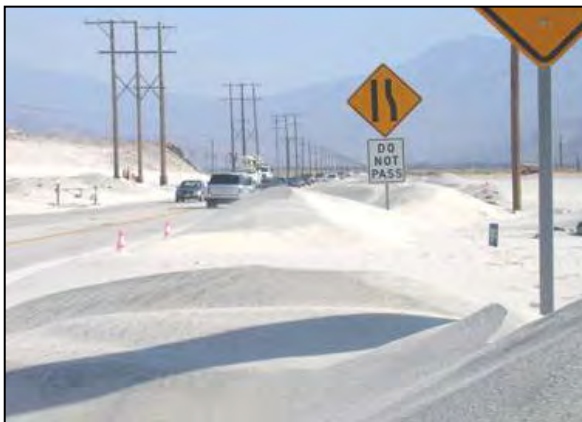
Windblown sand hazard along Indian Canyon Drive.
