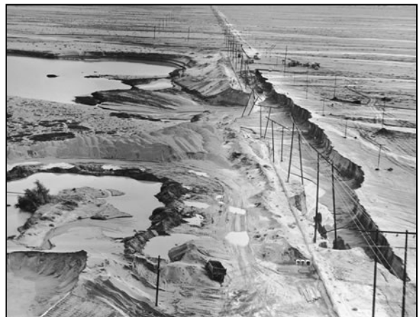
Flood damage to Indian Avenue by the 1965 Whitewater River floodwaters caused the road to be closed for 30 days, adding to the isolation of Palm Springs. (Source: RCFCWCD)
