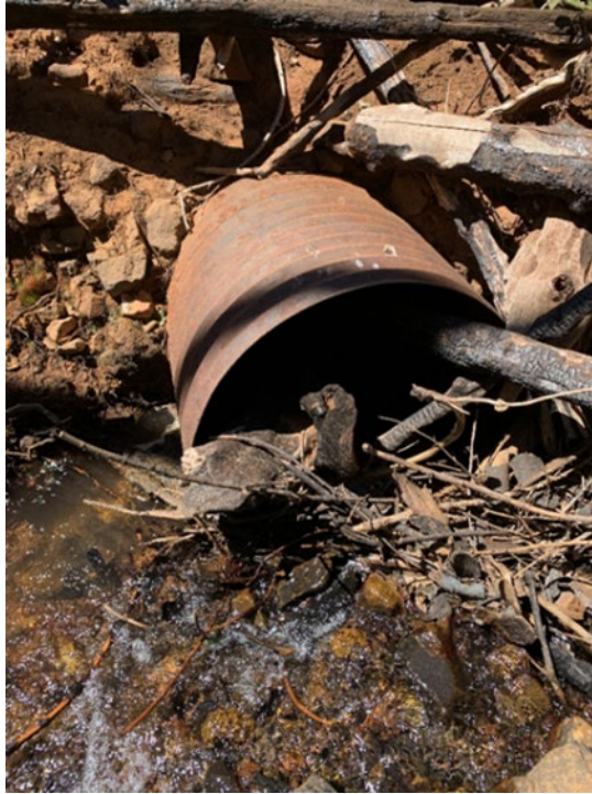
Figure 4. A culvert partially blocked by burned wood and debris in the 2020 North Complex Fire in Butte County, California. In this picture, the road is acting as a partial barrier and a sink for runoff, sediment, and debris.
