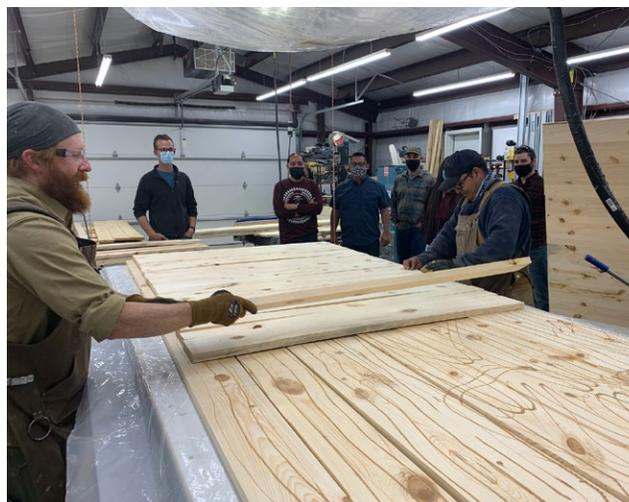
Manual layup of a CLT panel (Photo courtesy of TimberAge)
