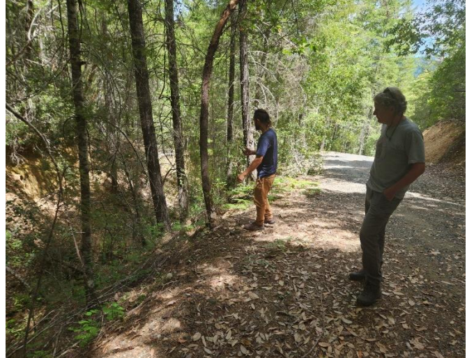
Figure 21. Colin looking at gully on Steve Brown's property where larger (4') post assisted check dams will be constructed.
