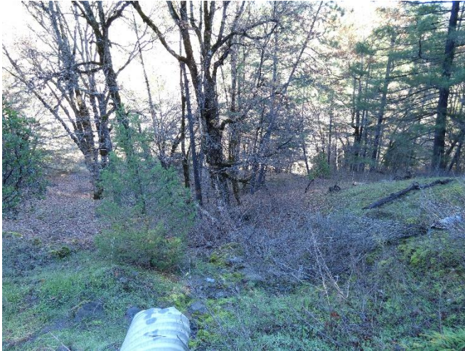
Figure 3. Culvert under Hargus Road with armoring at the outfall, but gully forming down-hill. 11/30/21.
