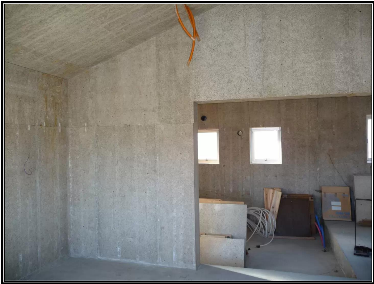
Figure 2.6 – Example Wood Strand Cement Board (WSCB) Used in Wall and Roof Applications (source Eltomation)
