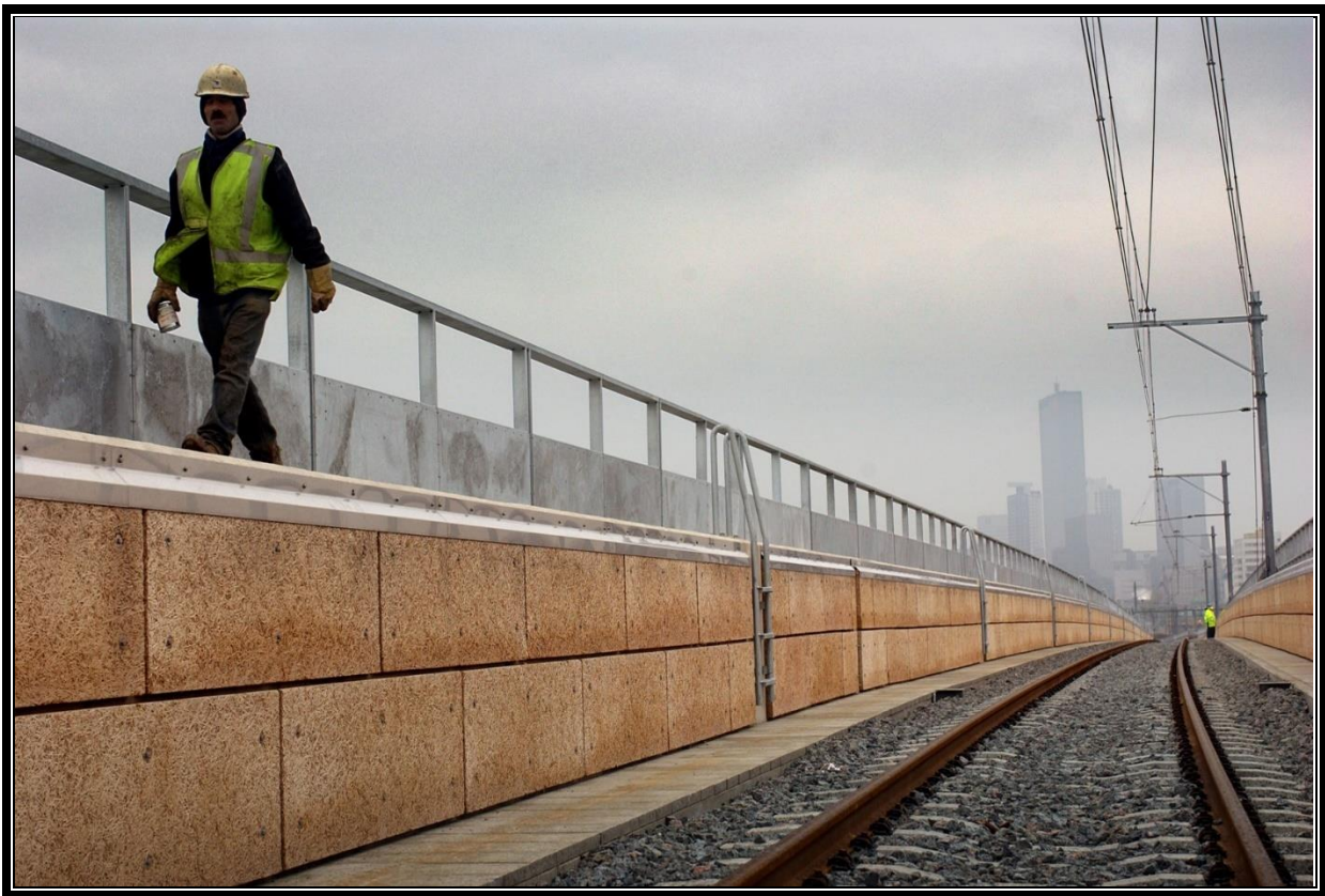
Figure 2.5 – WWCB In Use as a Sound Barrier Along a Train Track (source Eltomation)
