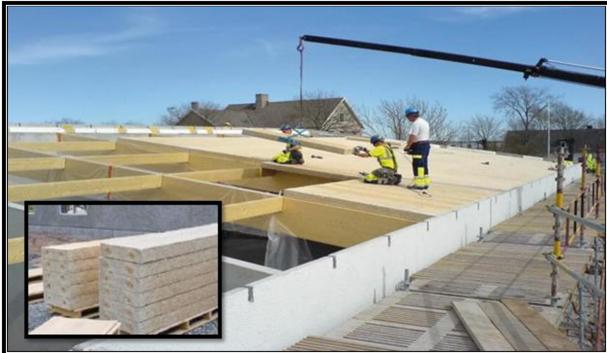
Figure 2.4 – Example of WWCB in Use as a Reinforced Roofing Panel (source Eltomation)
