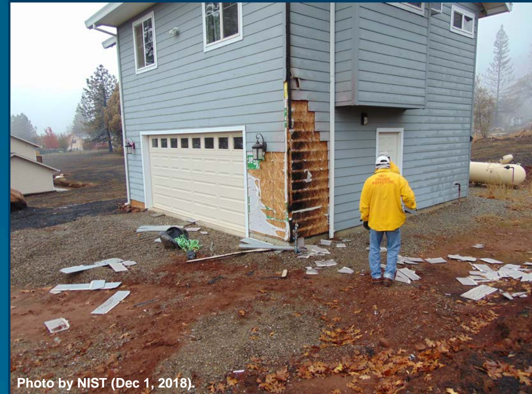
b) Associated evidence of the fire ignition and defensive actions encountered during NIST damage assessments.
