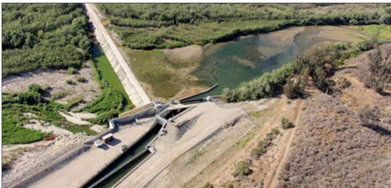
Figure 9-4. UWCD's Freeman Diversion
