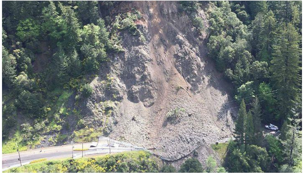
Figure 4-43: Landslide on Highway 101
