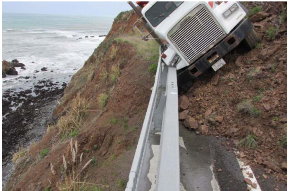
Figure 4-44: Mudslide on Highway 1 in Mendocino County Photo by The San Francisco Chronicle, https://www.sfchronicle.com/bayarea/article/Storm-watch-Scary-moments-as-landslide-takes-out-6884870.php#photo-9612874
