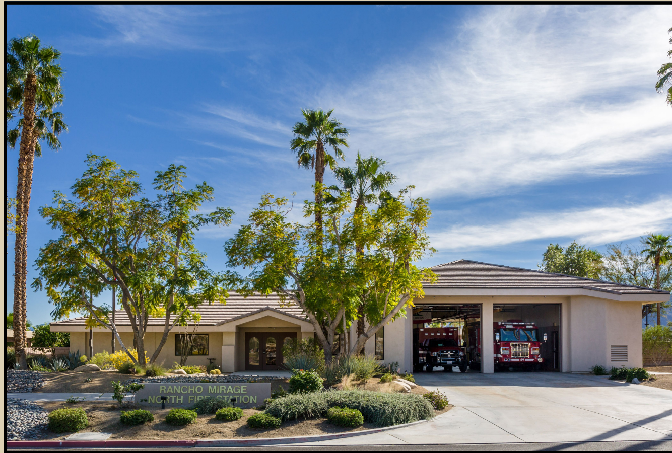
Rancho Mirage Fire Station 69.
