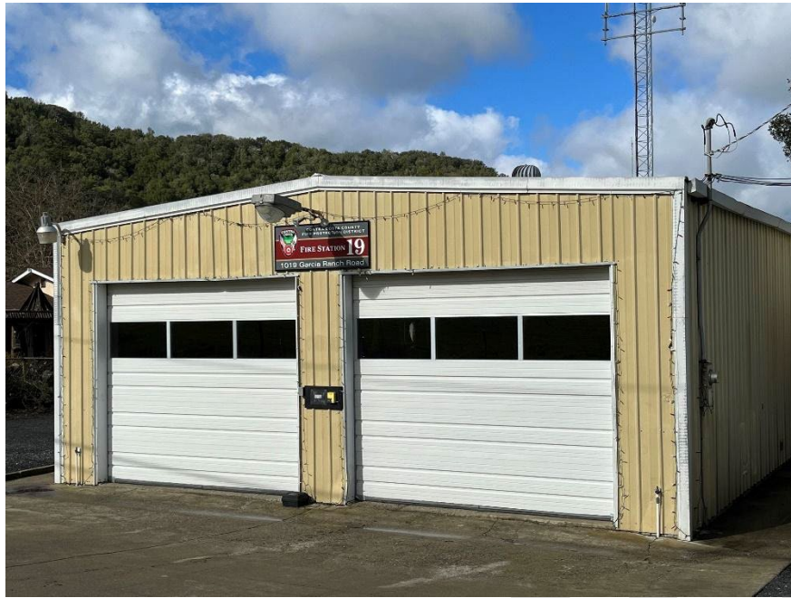
The Contra Costa Fire Protection District operates Station 19 in rural Briones Valley.
