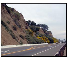
The instability of the Capistrano Bluffs is an ongoing concern. Regulations require that development be adequately set back from bluff edges, and traffic below must be protected from potential landslides.
