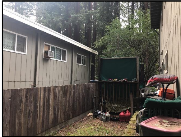
Figure 5: An example of a sampled 1038(c) where an adjacent parcel (left) had a structure and fuel in close proximity to the structure (right) that was the object of treatment under the submitted 150 Foot Exemption.
