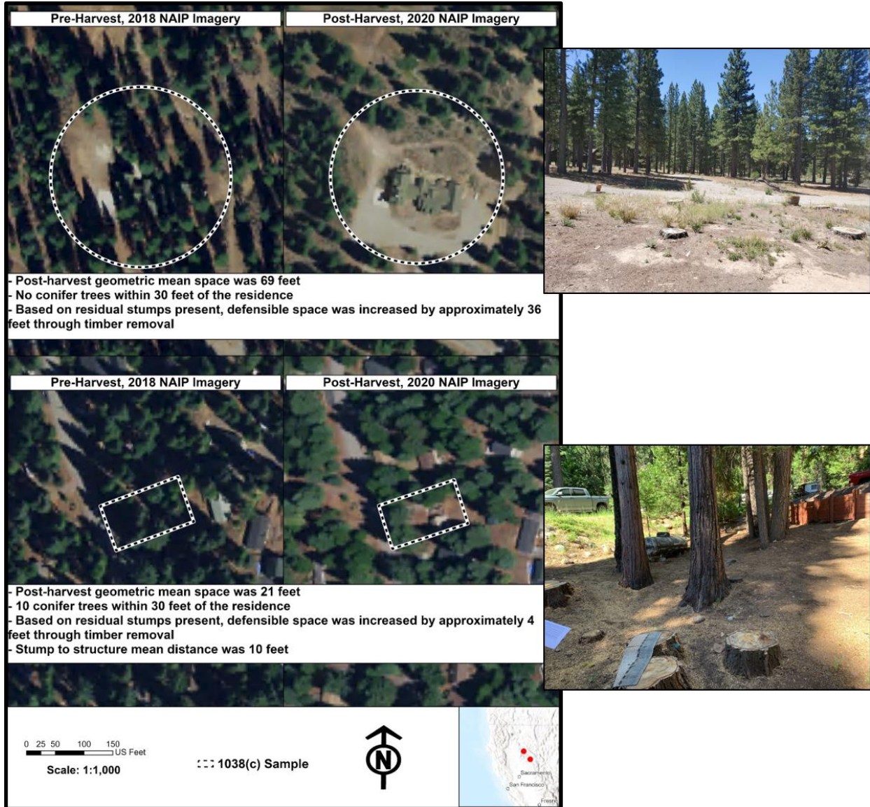
Figure 12: Top, an example of a 1038(c) that met all aspects of the intent of the 1038(c) Exemption, with the creation of over 30 feet of defensible space, single tree specimens within 30 feet of the residence, with pre- and post-harvest NAIP imagery, and a post-harvest image to the right shown. Bottom, a 1038(c) on a parcel less than one acre in size, that removed conifers from within 10 feet of a residence, however retained multiple trees within 30 feet, and had less than 30 feet of defensible space following operations, with pre- and post-harvest NAIP imagery and a post-harvest image to the right.
