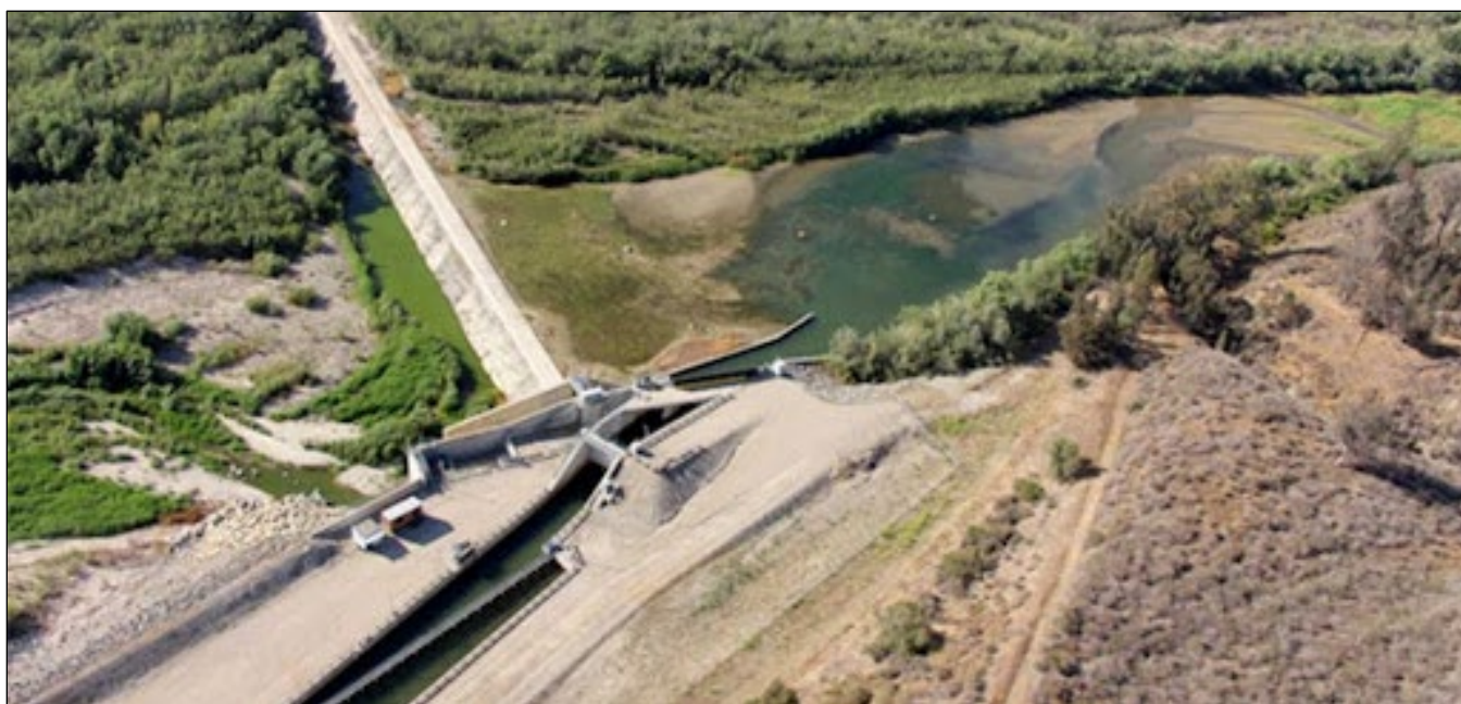
Figure 9-4. UWCD's Freeman Diversion
