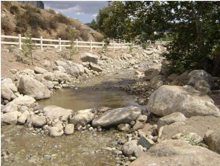
Yucaipa's stream restoration and landscaping projects recharge the aquifer, filter pollutants, and enhance water quality.
