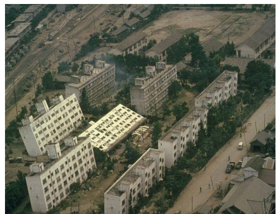
Liquefaction caused by the 1964 Niigata, Japan earthquake caused these apartment blocks to experience severe leaning. Image from the University of Washington.
