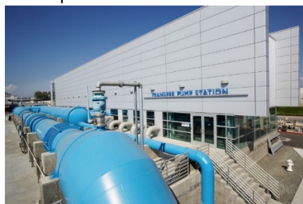
The Orange County Sanitation District treats Irvine’s wastewater. Image from IMEG.
