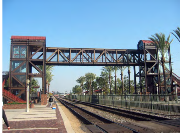
The pedestrian bridge over the tracks at the Fullerton Station. Image from PlaceWorks.
